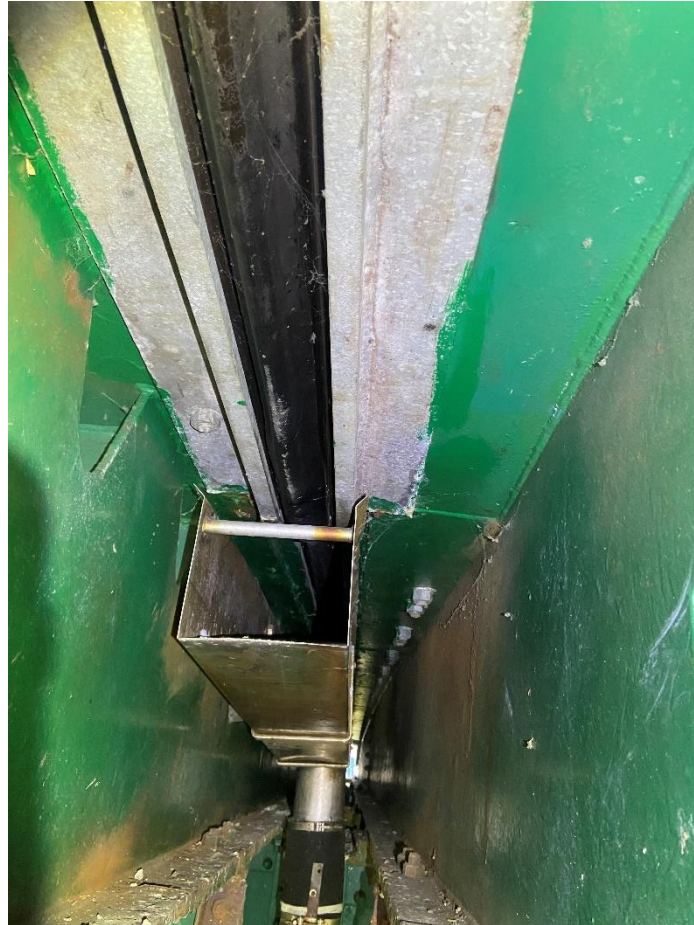
Figure 20: Typical Expansion Joint (Joint at Bent 19 Shown).
