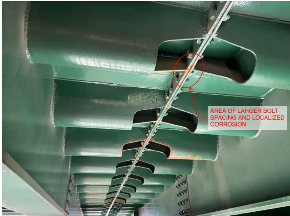
Figure 17: Typical OSPD Splice Condition (Splice 18A Shown).
