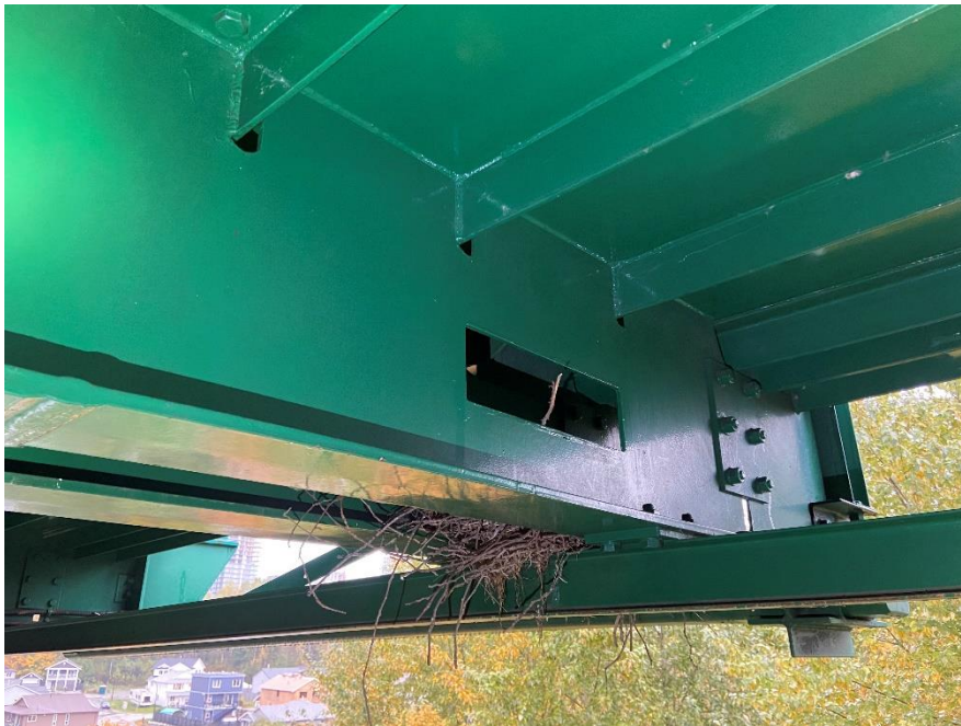
Figure 16: Typical Condition of Sidewalk Panel Plate Welds.
