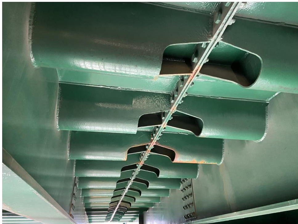
Figure 3: Typical OSPD Bolted Transverse Splice
