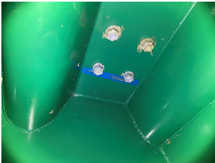
Figure 22: Cracked Paint at Expansion Joint at Bent 19 Identified Previous to this Inspection.
