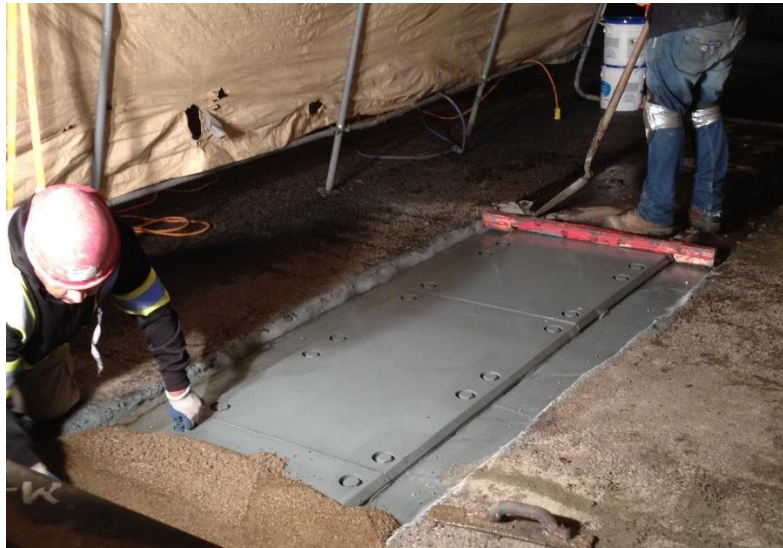
Figure 4: Link Plate Installed at Breather Joints in 2014 (BC MoTI)
