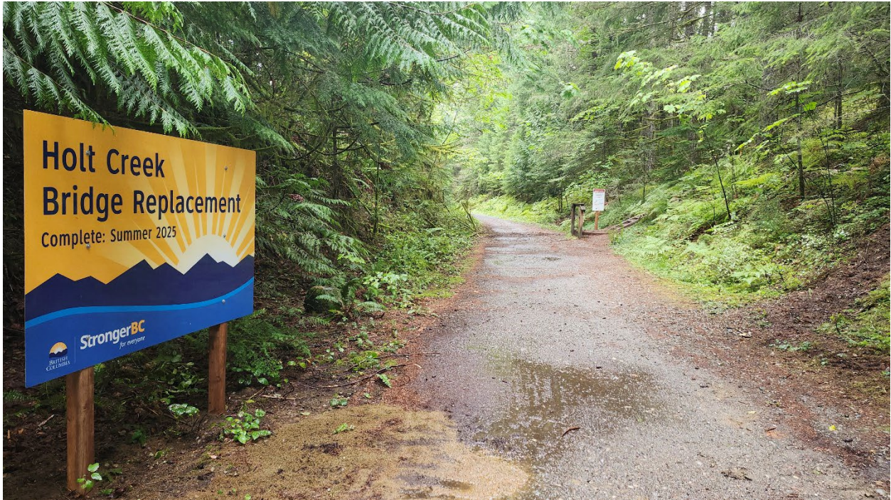
Holt Creek Bridge West Side
