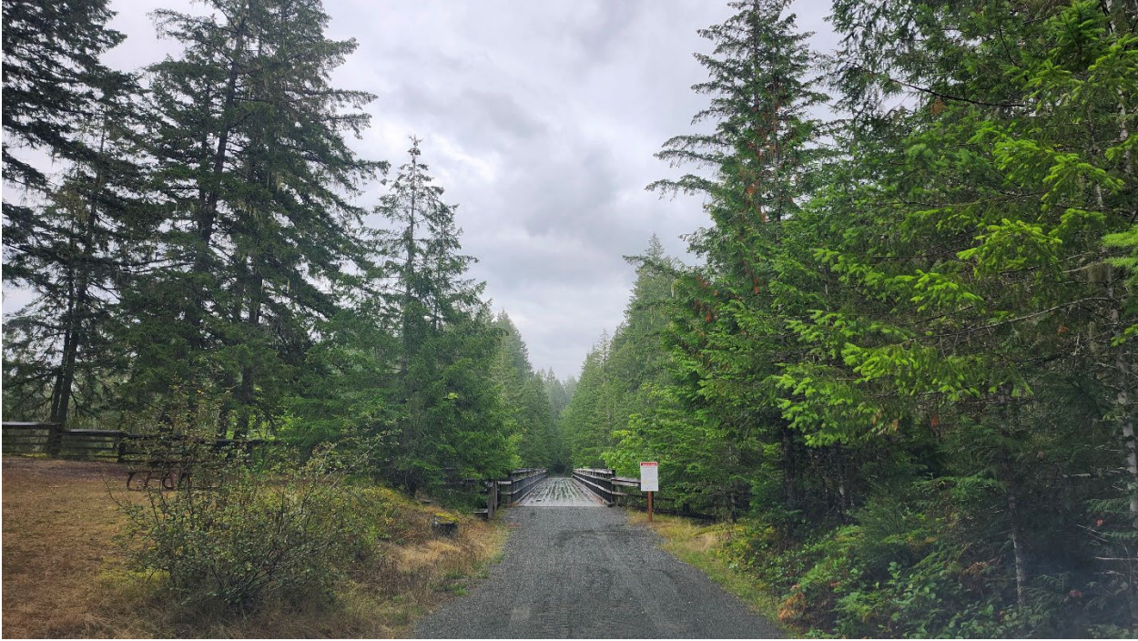
CVT Heading East to 66.2 Mile Trestle
