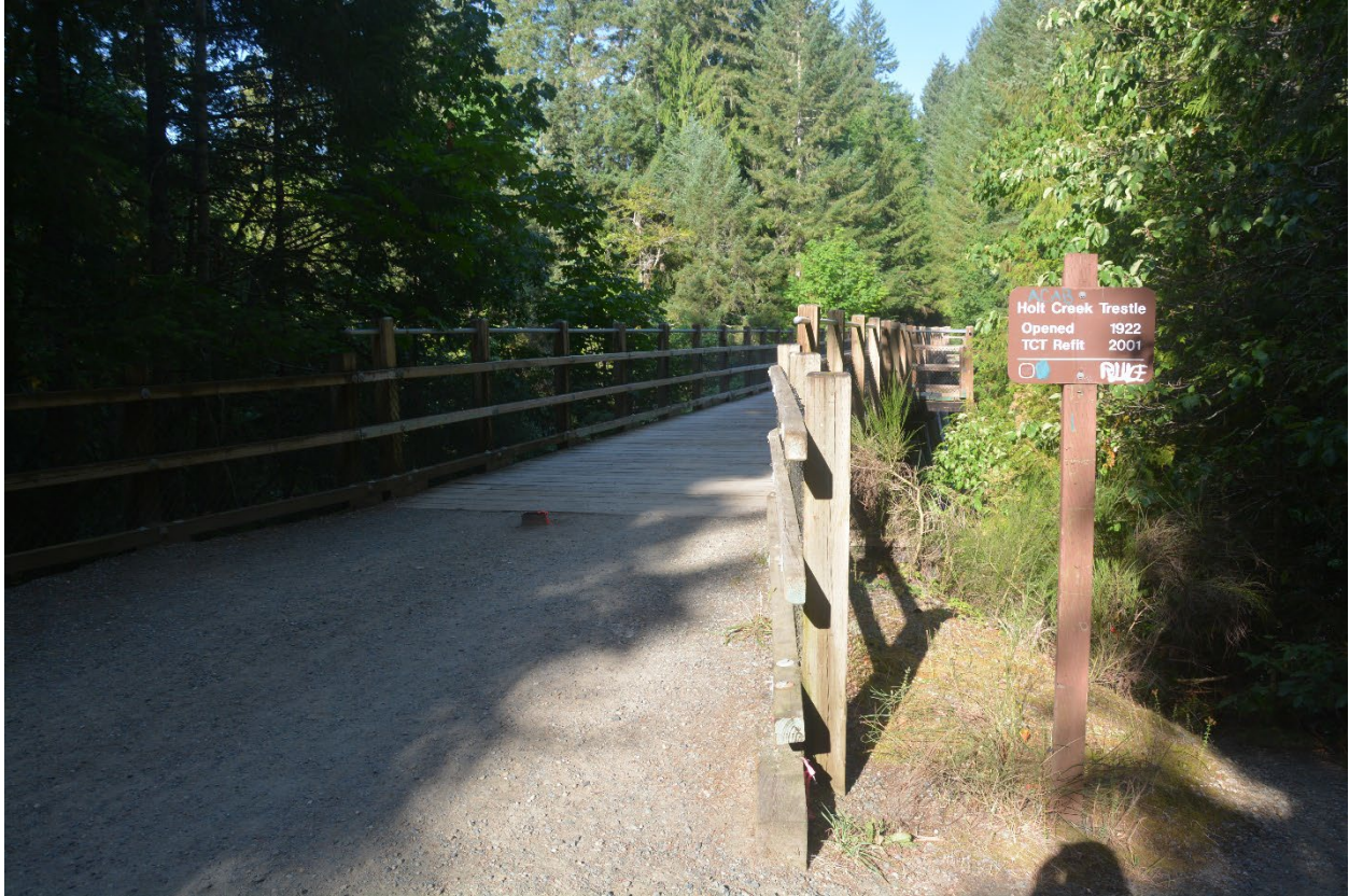
Holt Creek Bridge East Side
