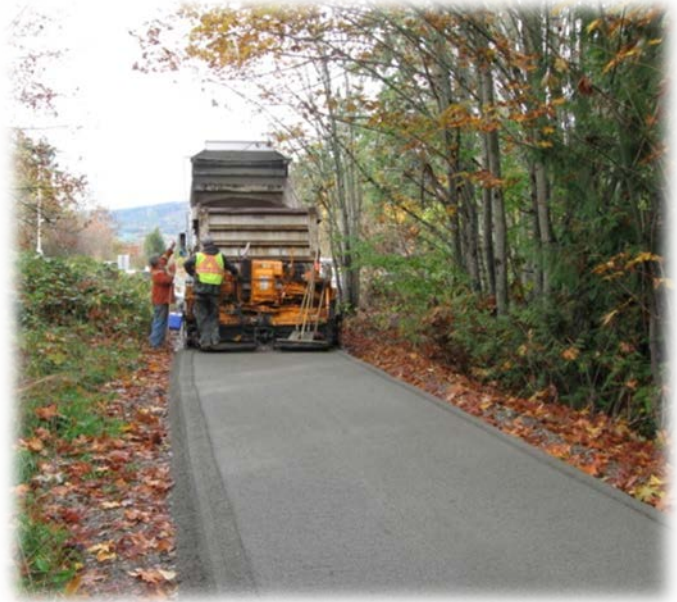
Surfacing the Cowichan Valley Trail
