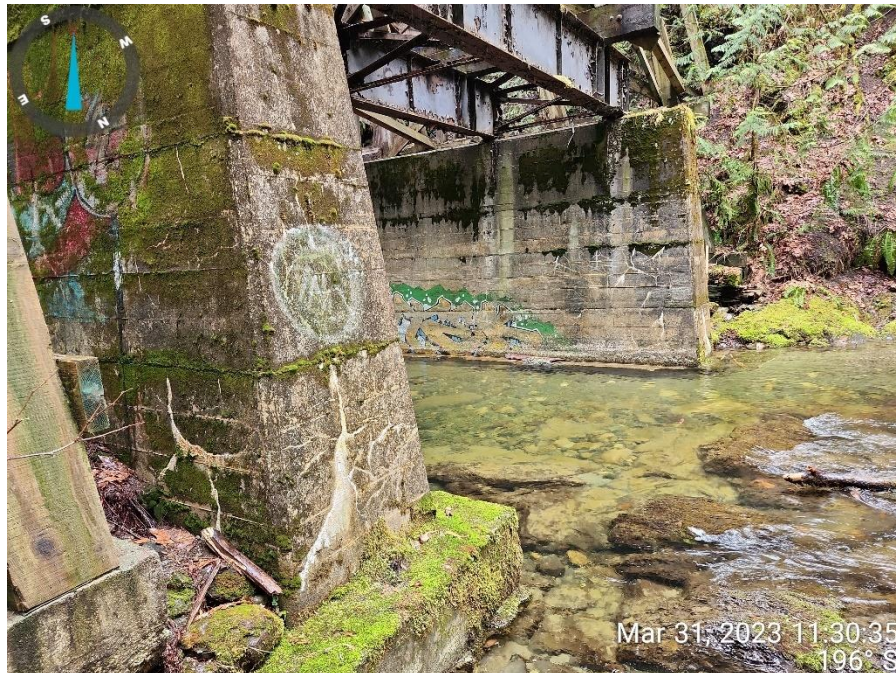
Photo 6 View of existing instream footings (to remain) Downstream Facing south.
