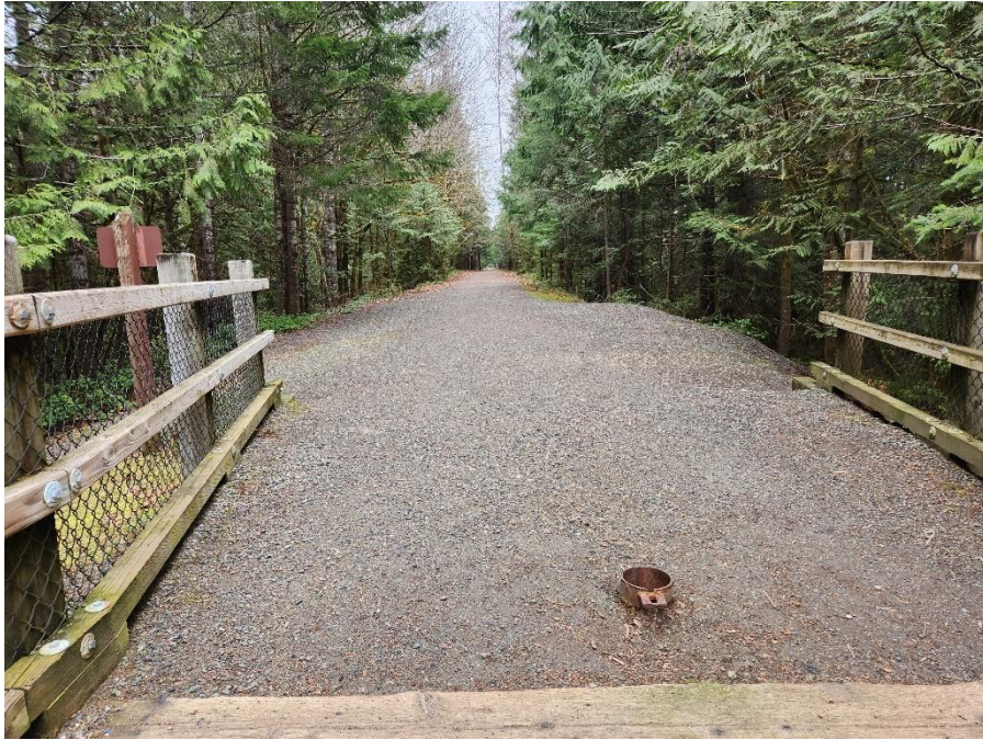
Photo 15 View of east access route. Facing east.
