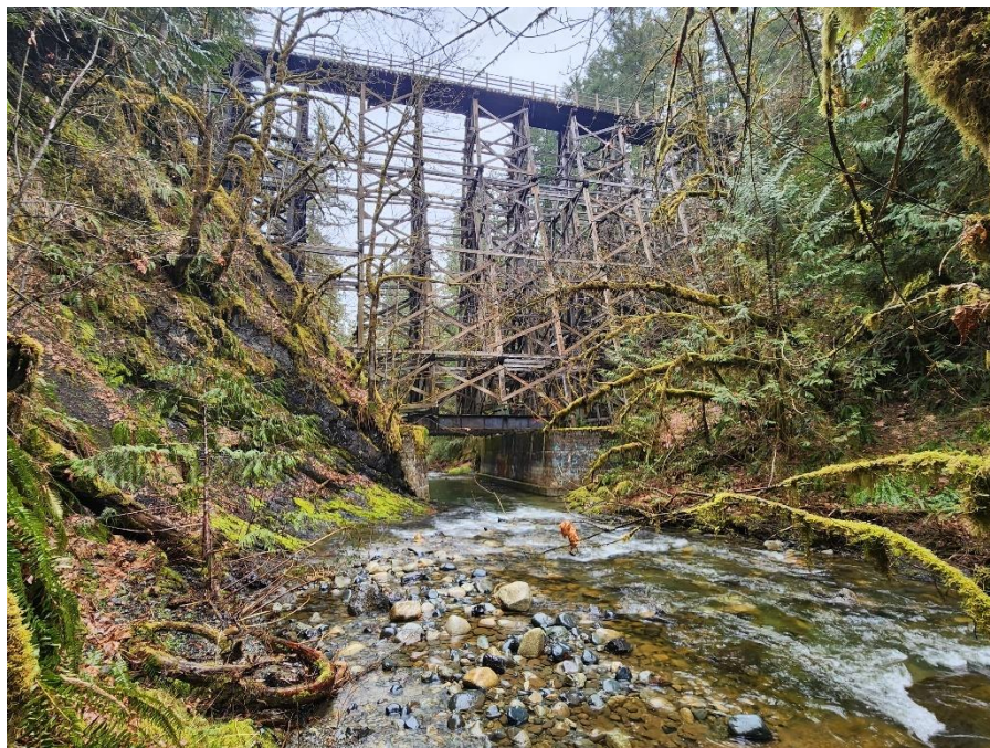
Photo 8 Existing wooden trestle to be removed. Facing south.
