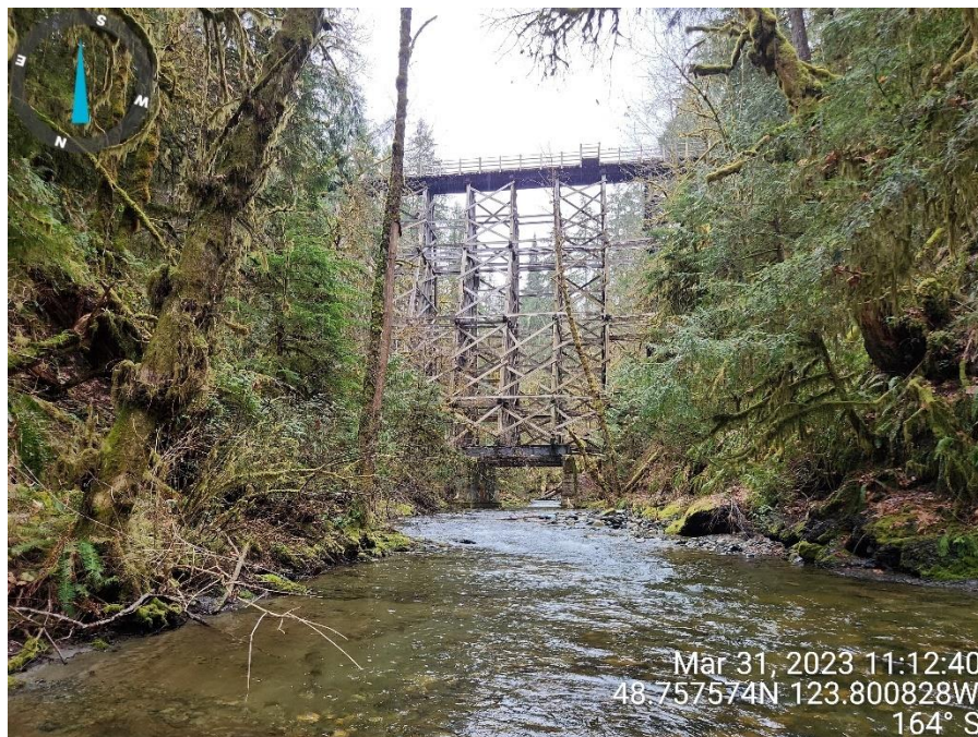
Photo 10 View of Holt Creek Bridge facing upstream (south).
