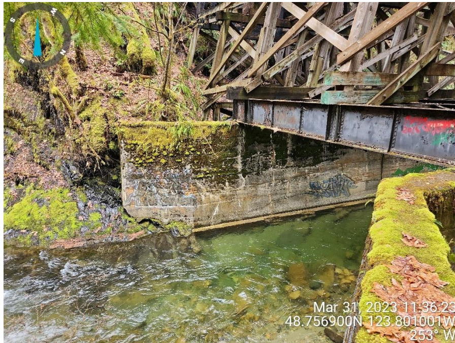
Photo 5 View of existing instream footings (to remain) Upstream facing west.
