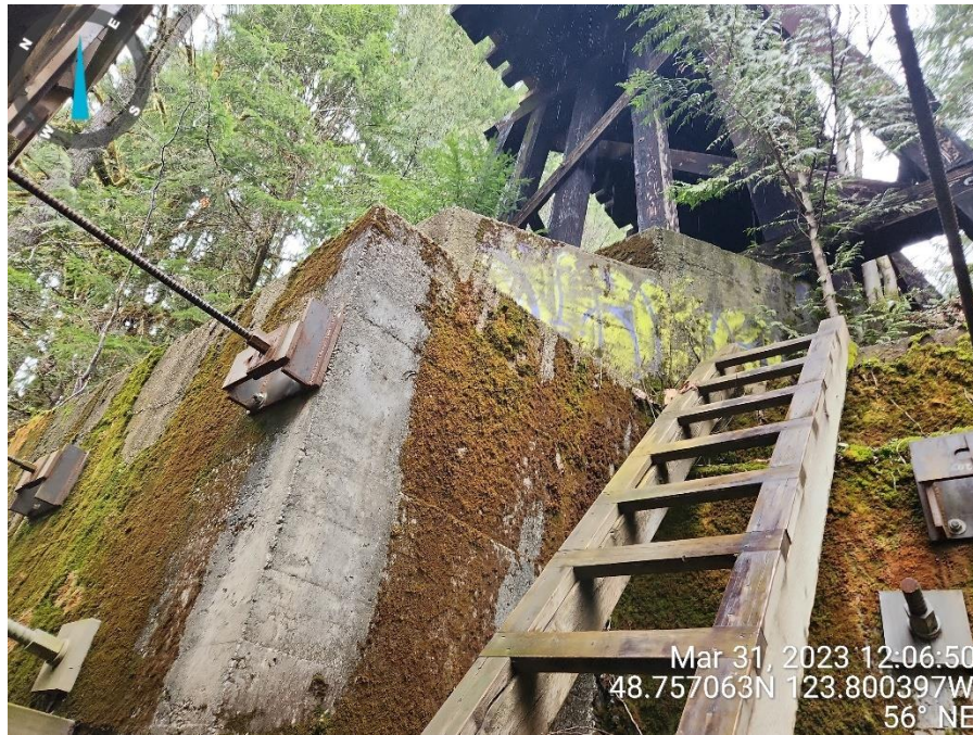
Photo 3 Existing eastern abutment supporting creosote timbers, Facing northeast.
