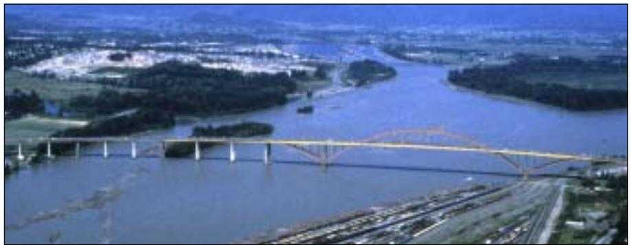
The Port Mann Bridge carries about 120,000 vehicles over the Fraser River daily. A fifth lane will be added to the bridge by moving the walkways to the outside of the metal arches and widening the concrete approach spans.
