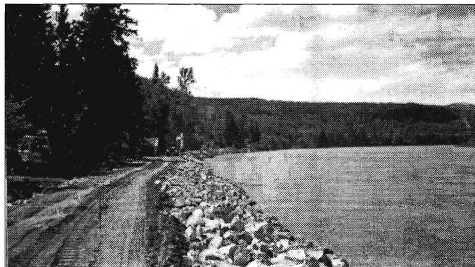
A highlight of Laurie's time in Terrace has been the construction of this dike beside the mighty Skeena River. The job involved 2,603 truck loads of riprap and cost more than \$280,000.
