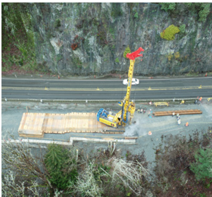
Image 10: Malahat Hwy restoration at Tunnel Hill
