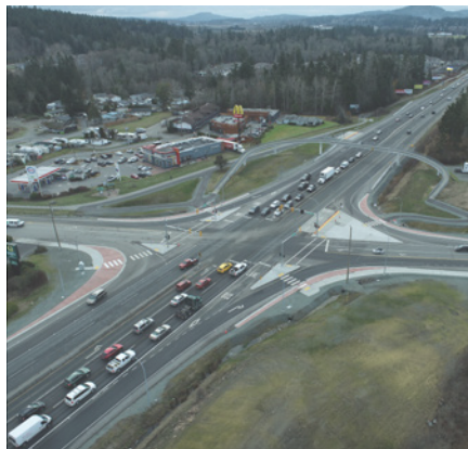
Image 2: Installed transit queue jumpers on Hwy 17 at Mt Newton Cross Road
