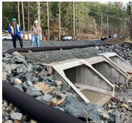
Image 11: Hwy 14 drainage improvements
