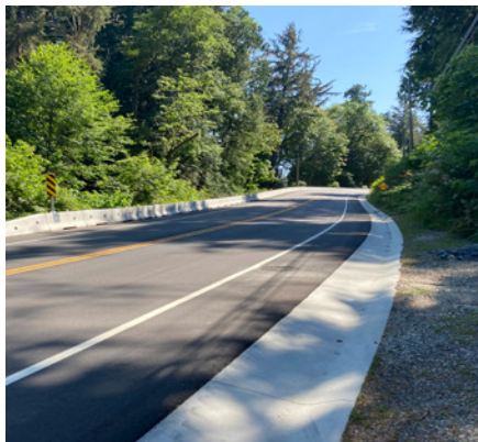
Image 7: Shoulder widening on Hwy 14 in Sooke
