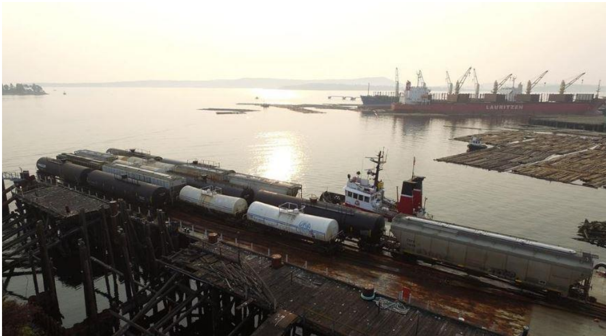
Figure 5: Rail Barge Slip at Wellcox Yard
