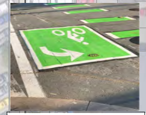
BIKE BOX (BB) TO BE LOCATED BETWEEN CROSS-WALK AND BIKE CROSSING (TYP.)
