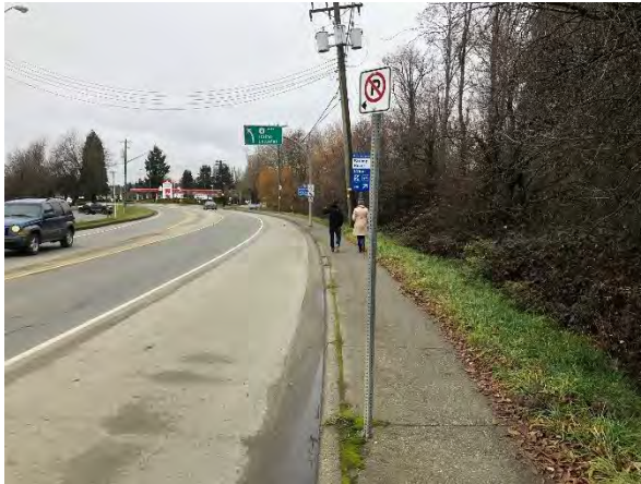
Highway 4 Looking West towards Beaver Creek Road
