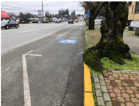
Root Structure Taking Over the Curb
