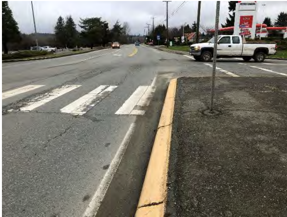
Highway 4 Marked Crosswalk with no Curb Ramp
