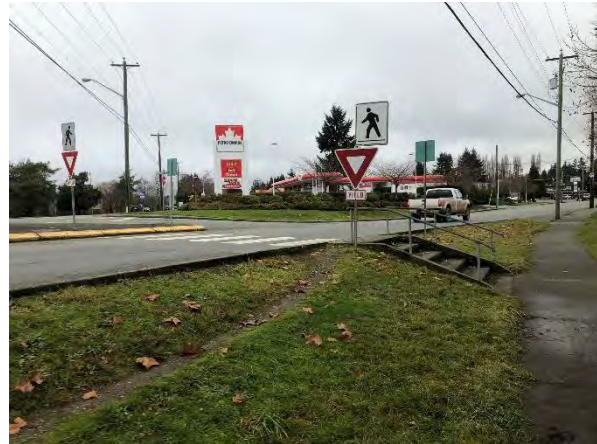
Inaccessible Crosswalk at Beaver Creek Road
