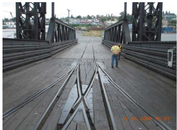
Barge Ramp in Nanaimo, north end of Wellcox Spur
