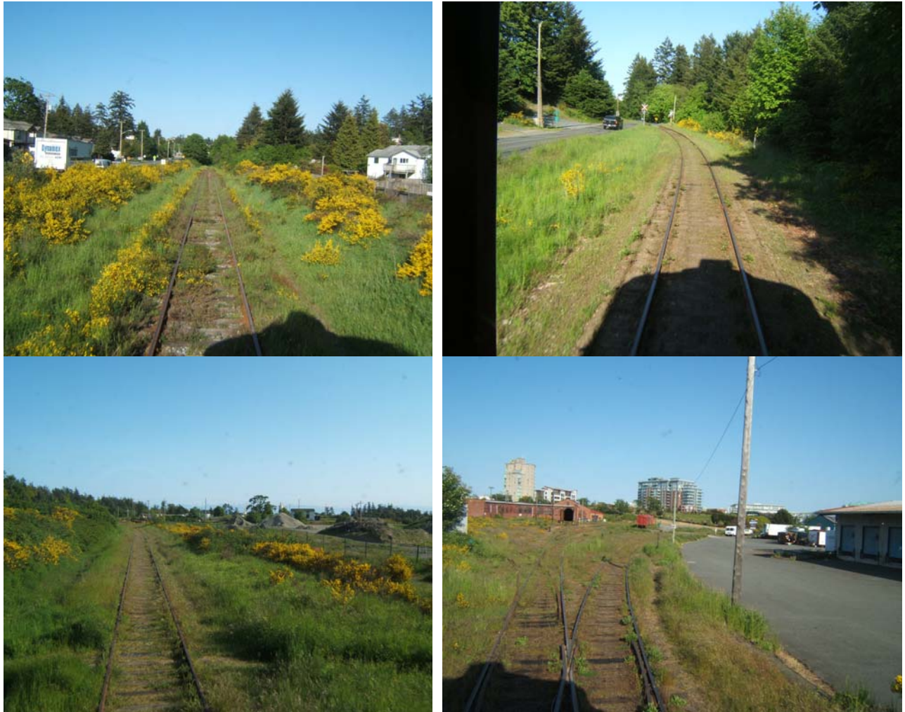
Illustrations (top): Overgrown track bed in Langford (left); Approaching Atkins grade crossing (right); and (bottom): Trackside growth in View Royal (left); weed infestation at spur line to roundhouse (right).
