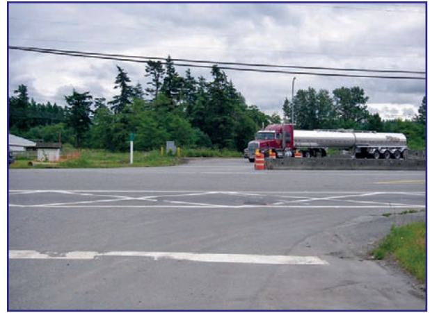
Northbound Weigh Scale Exit (Before)
