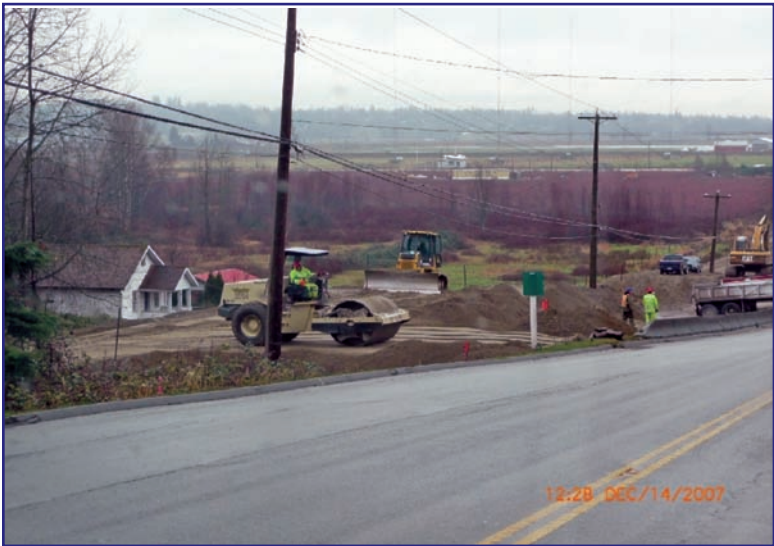
Final Lift of preload at the Archaeological Site
