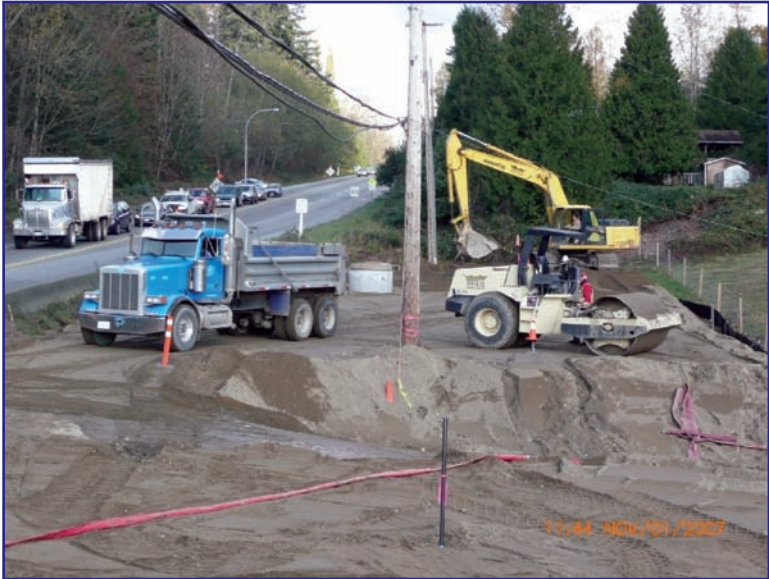
Stage two preload placement at the Archaeological Site
