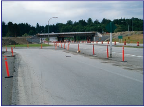
Highway 99 Facing South – New Bridge
