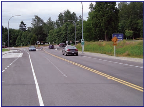
West Roundabout Facing South (In operation)
