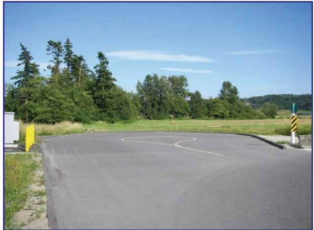
Turnaround Facility behind Northbound Weigh Scale Exit
