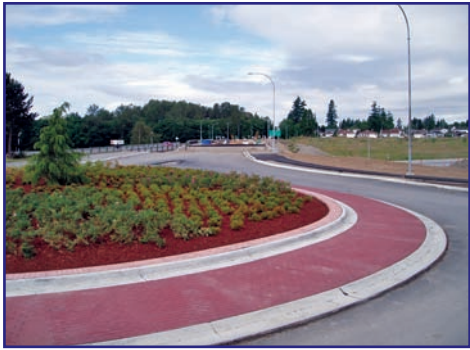
East Roundabout – Bridge in Background
