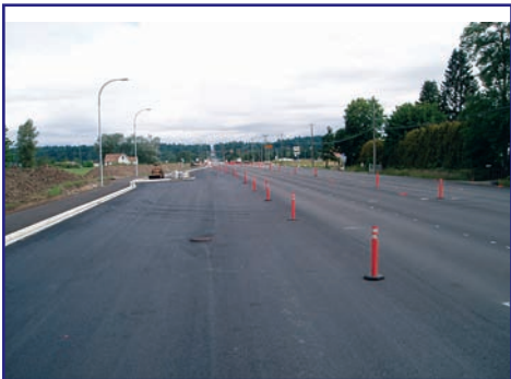
176th Street South End of Project Facing North
