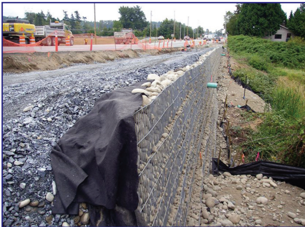
West Retaining Wall (During Construction)
