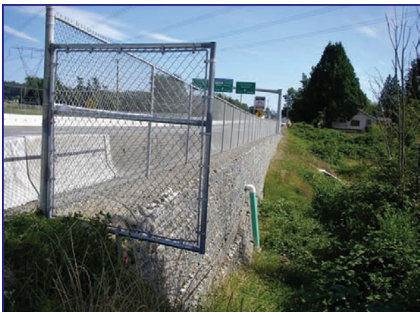
West Retaining Wall (Completed)
