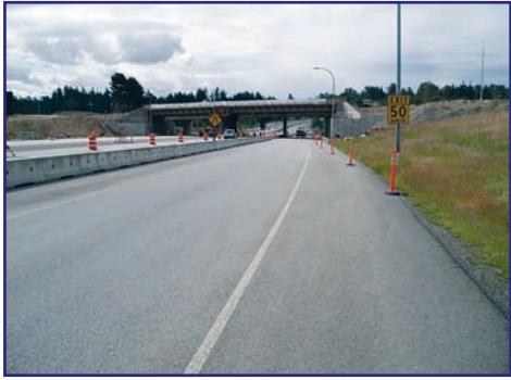
Highway 99 Facing South – New Bridge
