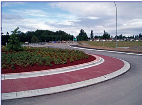
East Roundabout – Bridge in Background
