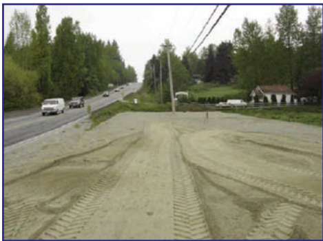
Northern extents of Highway 15 Project Preload
