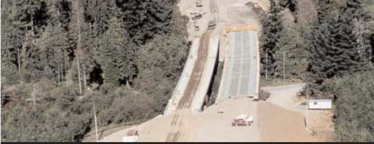
Morrison Creek Bridge on Vancouver Island Highway Project
