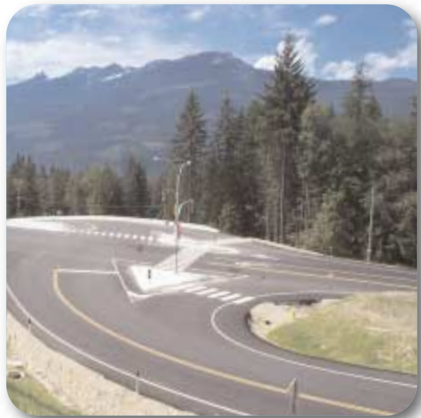
Construction of the Nakusp Bypass in the Kootenays is one of BCTFA's investments to improve mobility in the North and the Interior
