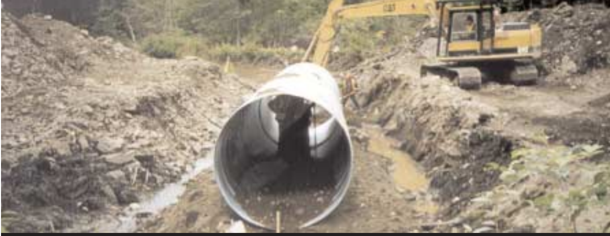
Installation of fish passage culvert as part of Nisga'a Highway improvements
