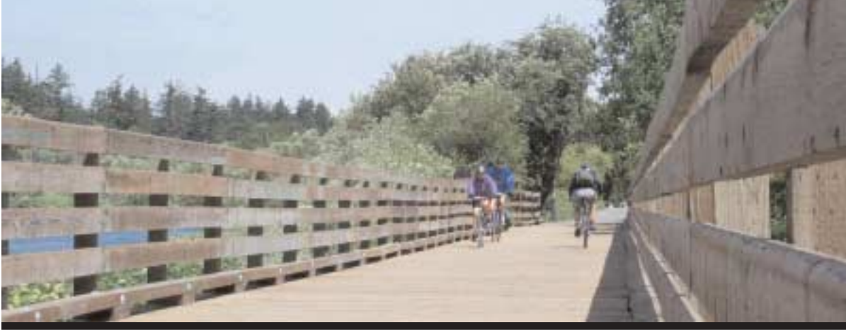
Construction of the Blenkinsop Bridge and its approaches was assisted by CNP funding
