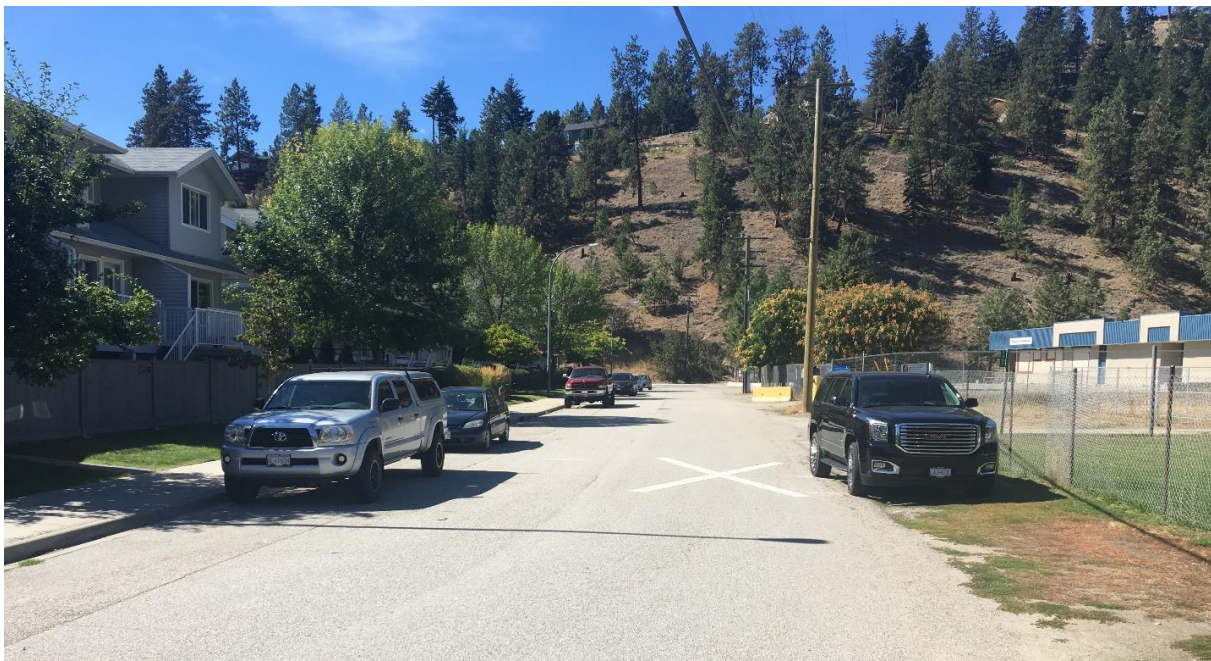
Figure 4.2: Traffic from Chidley Road will be Rerouted Along Clements Crescent and Pass by Peachland Elementary School (Right)
