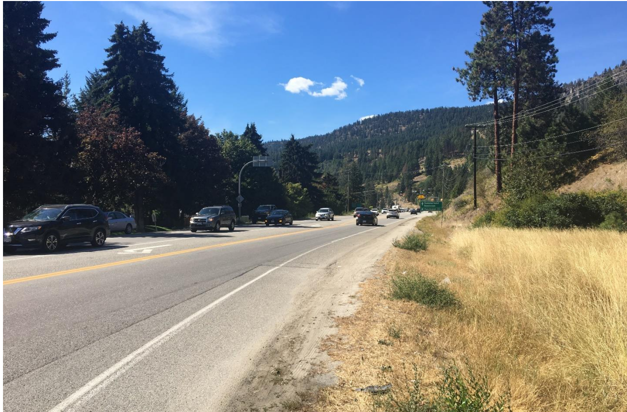
Figure 3.10: Highway 97 Looking South from Clements Crescent to Ponderosa Drive
