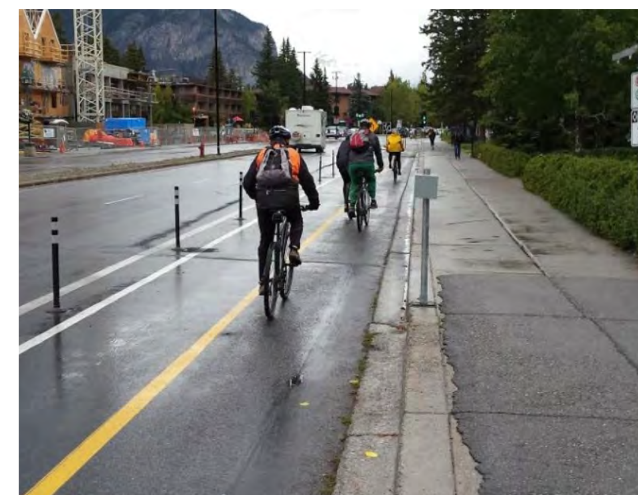
Separated bike lane on Banff Avenue in Banff. Image from: cbc.ca
