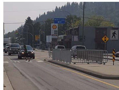
Mid-Block Pedestrian Crossing
