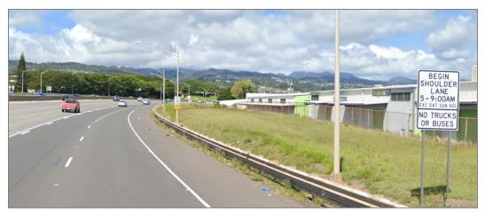
Figure 3.5: Example of an AM Peak Hour Hard Shoulder Running System in Honolulu, Hawaii
