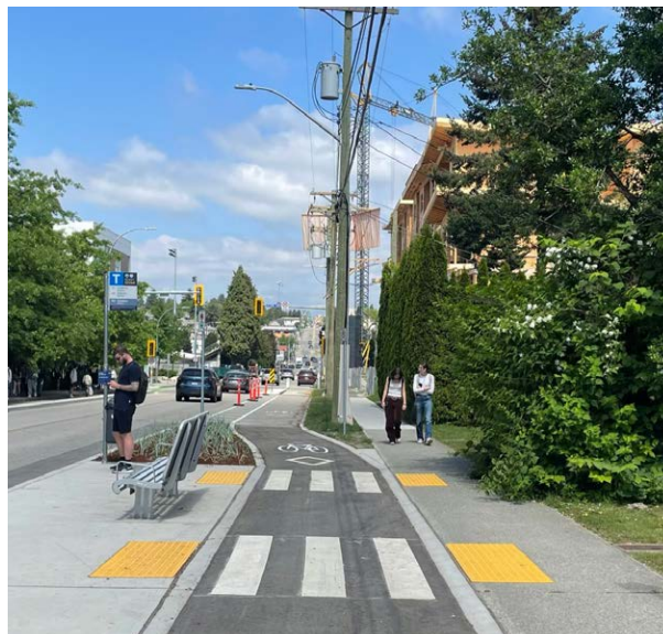
Figure 11: Detectable ‘Bookend’ at End of Island Platform Using Vegetation, New Westminster, British Columbia
