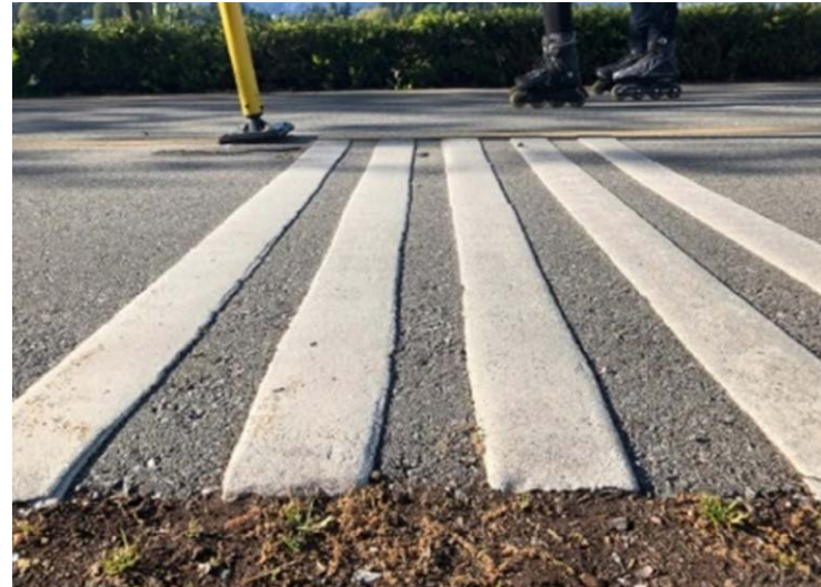
Figure 26: Example of Transverse Thermoplastic Pavement Markings, Vancouver, British Columbia
