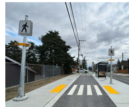
Figure 37: Actuated Flashing Beacon at Island Platform Crosswalk, Mission, British Columbia
