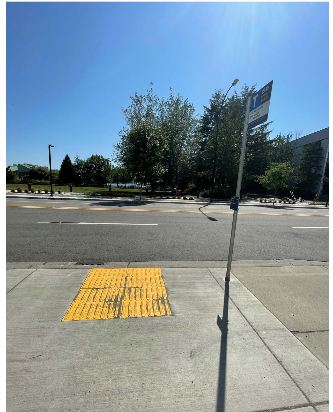
Figure 6: Bus Stop ID Pole and Tactile Directional Indicator Mat, North Vancouver, British Columbia
