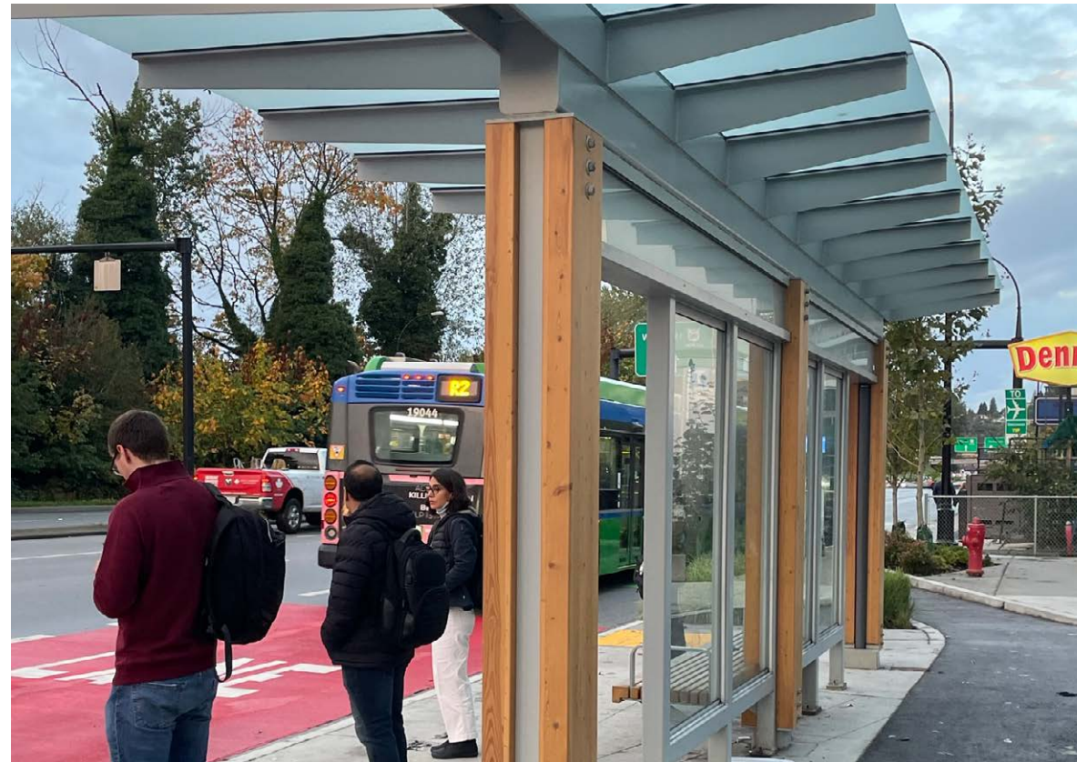
Figure 41: Example of Bus Shelter with No Side Panel and Clear Back Panels, North Vancouver, British Columbia
