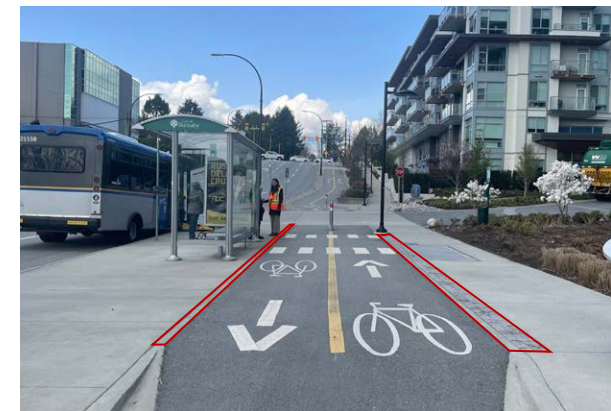
Figure 31: Examples of Edge Treatments that are Not Reliably Detectable, Burnaby, British Columbia (left) and Vancouver, British Columbia (right)
