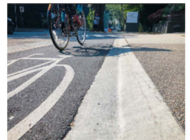
Figure 29: Intermediate-height Cycling Infrastructure with Beveled Curb, Vancouver, British Columbia
