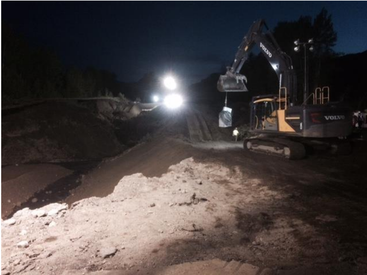
Figure 3-5 Nighttime Repair Work at Commotion Creek – June 2016
