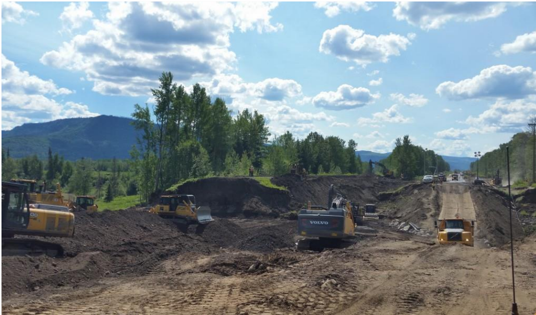
Figure 3-4 Road Repairs at Commotion Creek – June 2016
