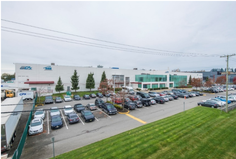
Figure 8.2-A: Surrey Distribution Center Exterior
