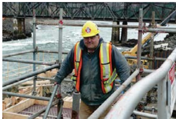
Ktunaxa Nation worker on the job at the Waneta Expansion Project.
