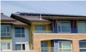
The Oliva building in Delta’s Tsawwassen Town Centre. Note the panels on rooftop for solar-assisted hot water heating.
