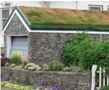
Green roof on single family garage in Victoria.
