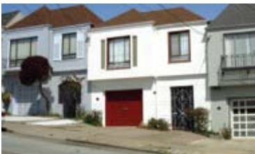
Example of row housing that could fit in a main street setting.
