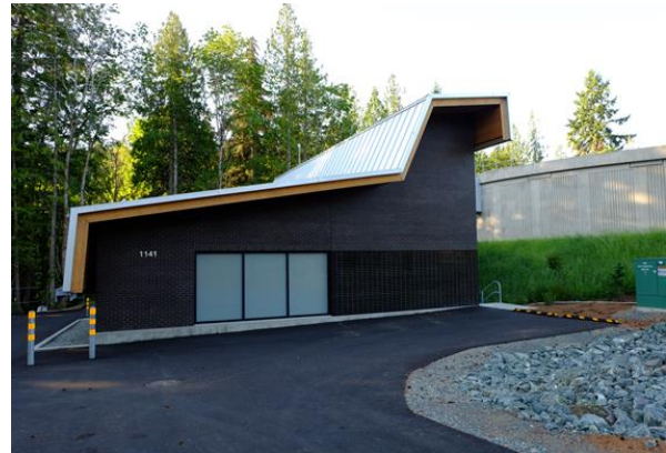
The City of Nanaimo's Energy Recovery Facility (image courtesy of the City of Nanaimo)
