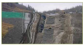
Gabions under construction in waste disposal area
