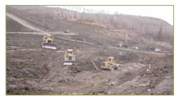
Construction/Placement of fill in the engineered waste disposal area
