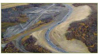
Substantial Completion (Aerial): Engineered waste disposal and new alignment; Partial old alignment at bottom left of the picture
