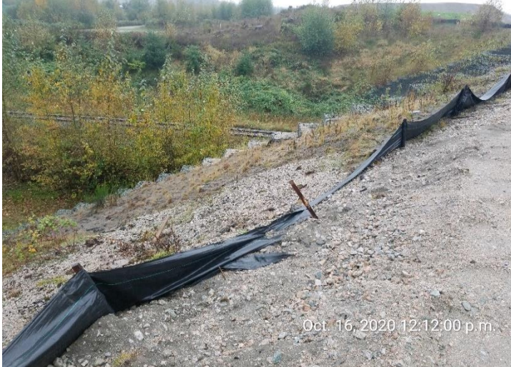
Photo 7. Portion of damaged silt fencing at the south end of Area D, adjacent to Highway 17.
