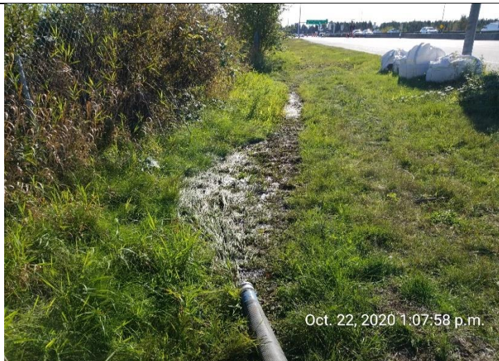
Photo 13. Dewatering into vegetated areas to prevent scour and allow for bio infiltration.
