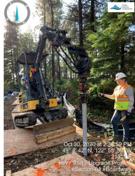
Photo 20. Installation of helical piles for the new boardwalk section in the Delta Nature Reserve.
