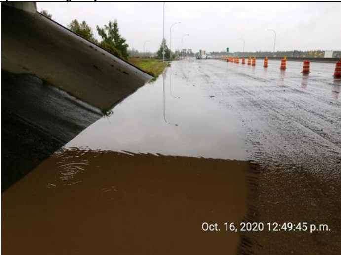
Photo 9. Sediment accumulation on pavement near Area G was contributing to sediment laden water.
