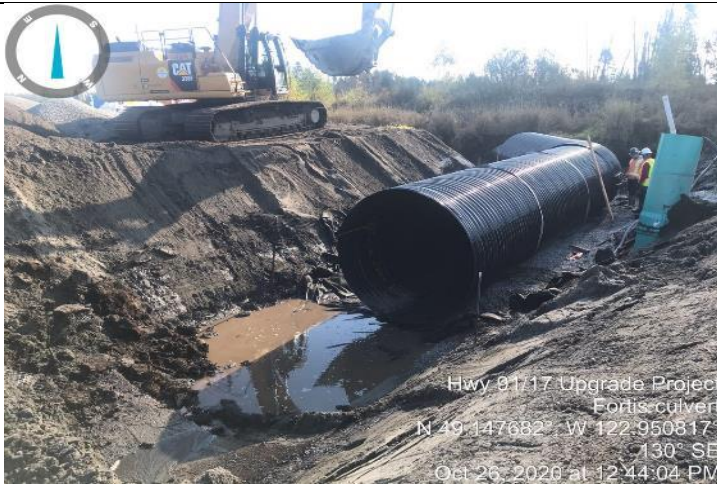
Photo 23. Installation of 2200 mm culvert over the Fortis line post fish salvage.
