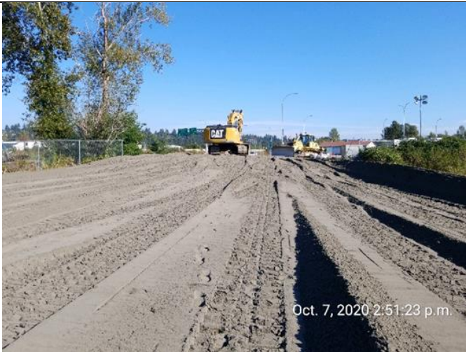
Photo 5. In general, most areas were stable due to placement of preload sand.
