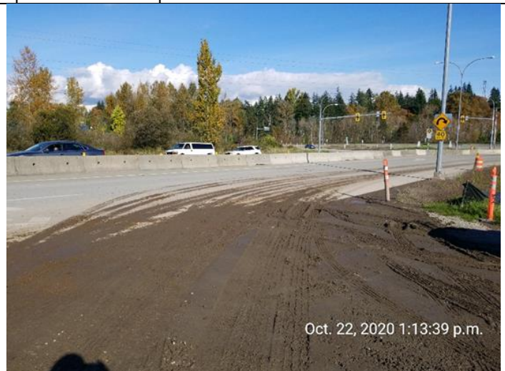
Photo 14. Track out was observed onto public roadways (Highway 91 offramp to Nordel Way).
