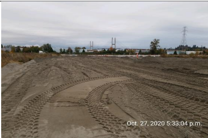
Photo 21. Most areas were covered with pre-load sand and were not considered to be erodible.
