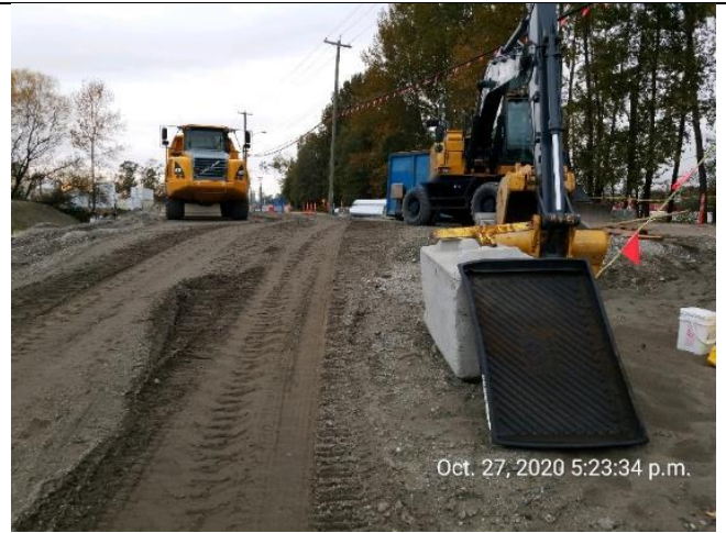
Photo 24. Although readily available, drip trays were often not placed under idle equipment.
