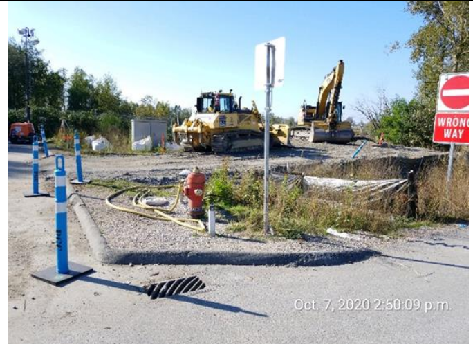
Photo 4. Unprotected CB at the Truck Stop (Area F) near an active access point.
