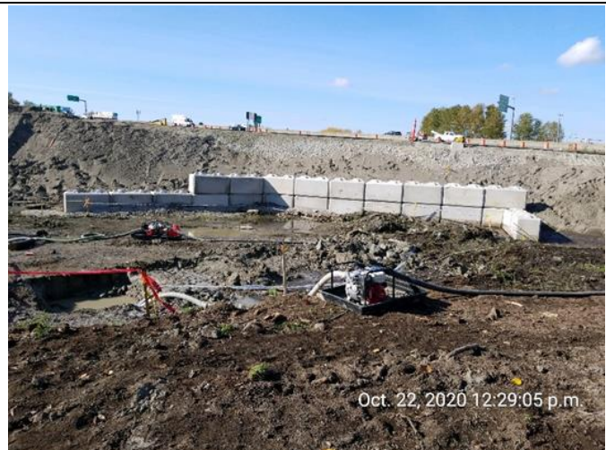
Photo 18. Lock block retaining wall at W01 detour.
