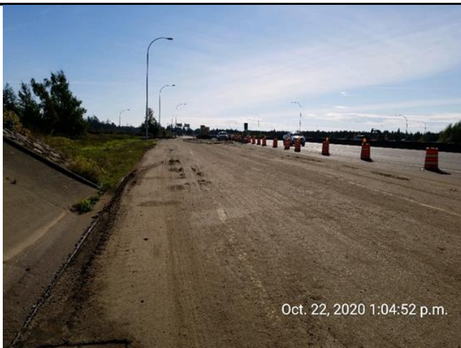
Photo 15. Sediment accumulation on pavement near Area G was contributing to sediment laden water. During periods of rain.
