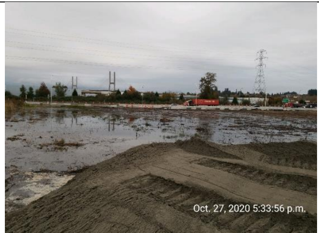
Photo 22. Low-lying areas throughout the project were filling with water due to a high-water table and increasing seasonal rains.
