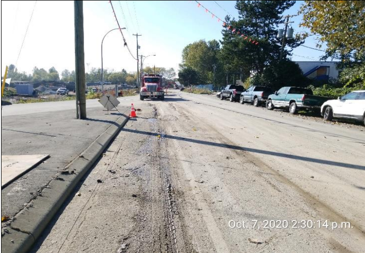
Photo 3. Some sediment accumulation observed on paved surfaces near Area C. Pavement is swept at the end of each day.
