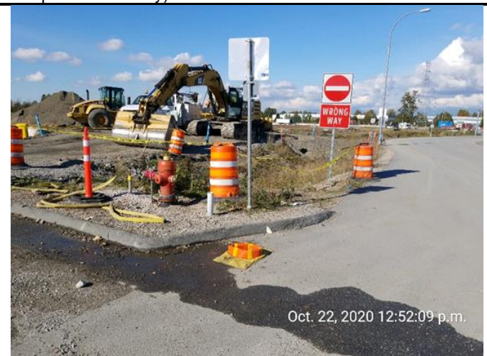
Photo 16. CB inserts had been installed at the truck stop.
