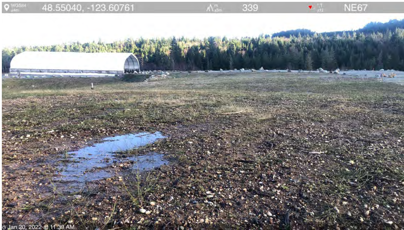
Photo 7: View of standing water on the southern portion of the PEA cap looking northeast (January 2022).
