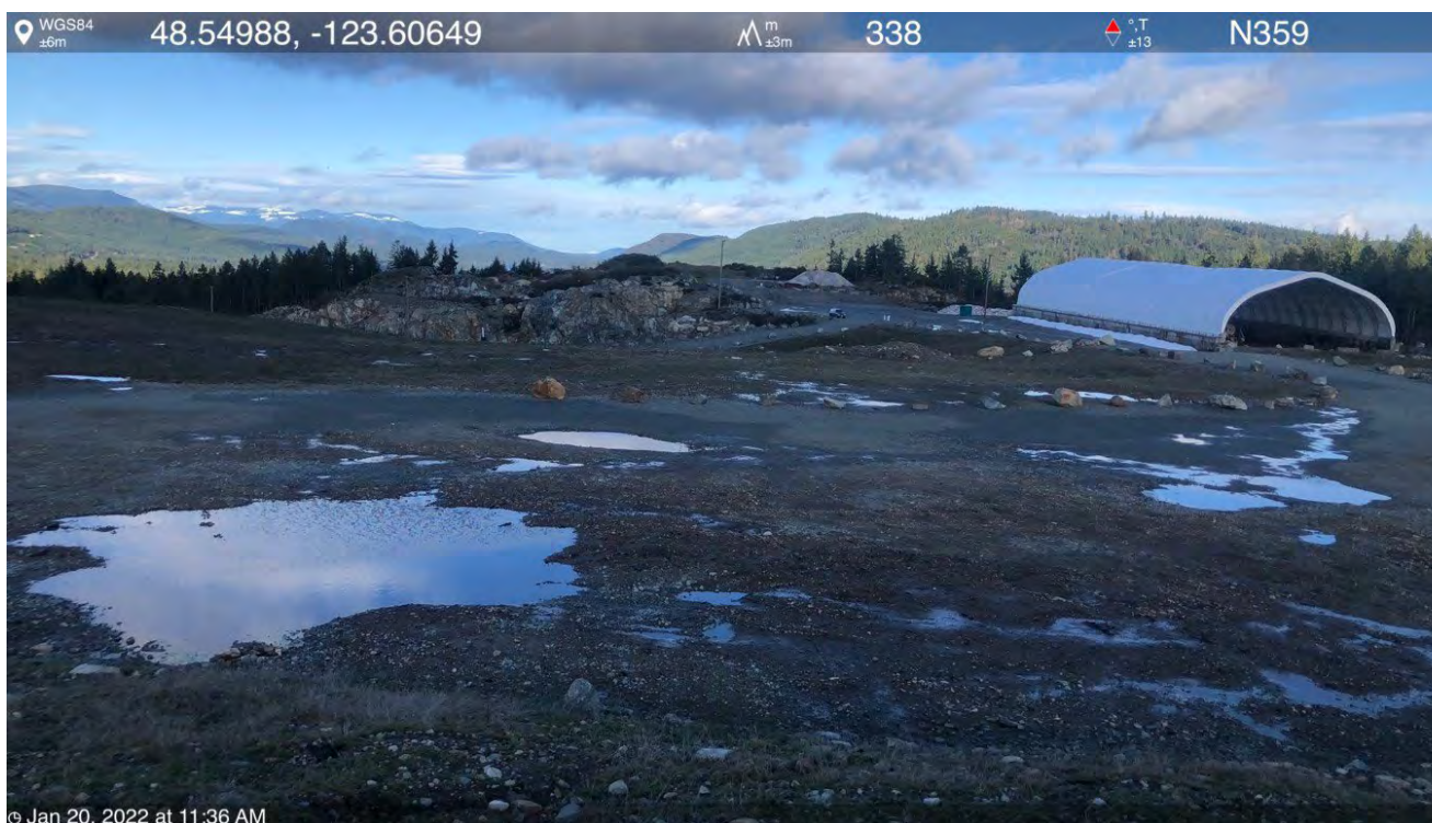
Photo 11: View of standing water at the south/southeast perimeter of the landfill looking north (January 2022).
