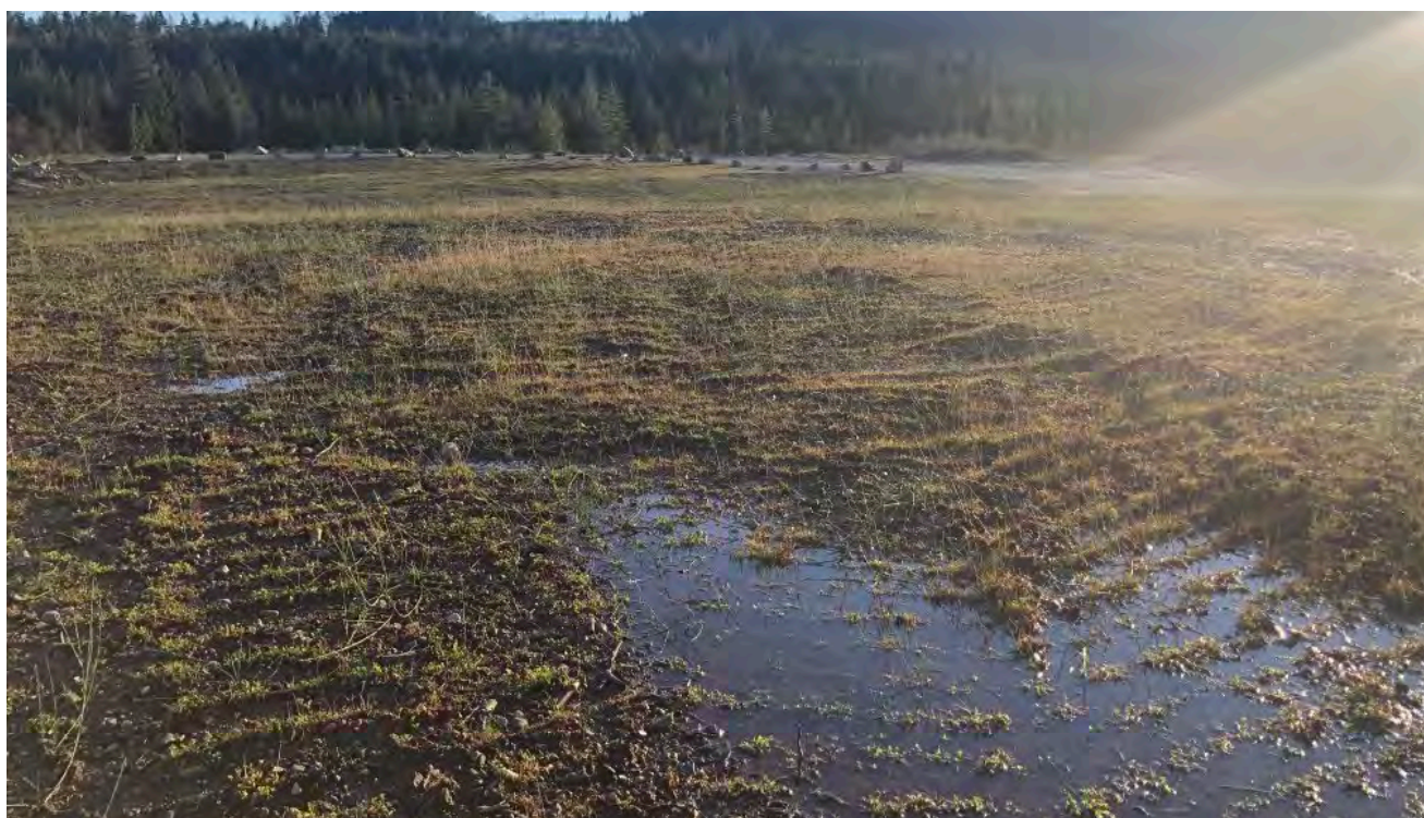
Photo 6: View of standing water on the southern portion of the PEA cap looking east (November 2021).
