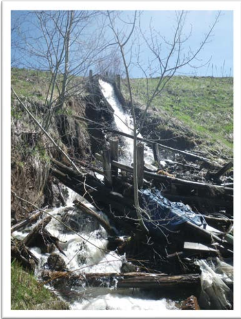
Photo 3: Myren Creek – collapsed flume and eroded dam face.
