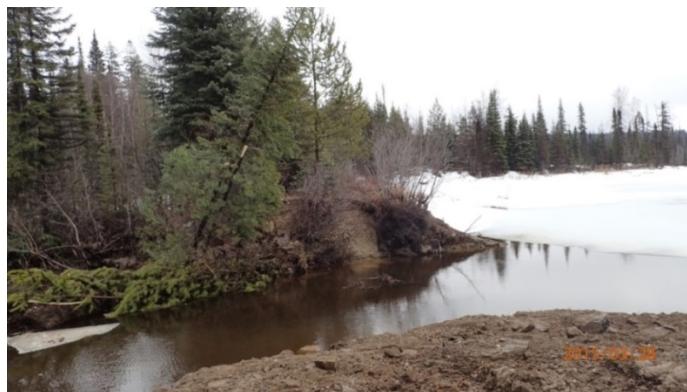
Photo 2: Embankment dam failure near Bear Lake, Regional District of Fraser Fort George
