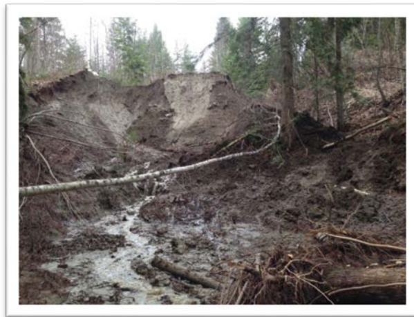
Photo 1: Embankment dam failure near Salmon Arm
