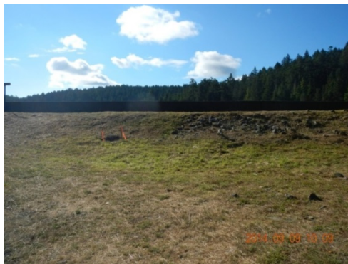
Photo 8: Butchart Lake Dam #5 – sinkhole on downstream face
