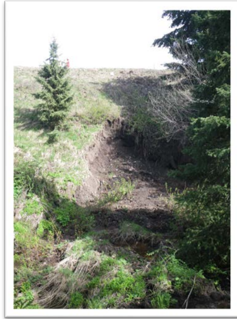
Photo 4: Myren Creek – slump on downstream face of dam
