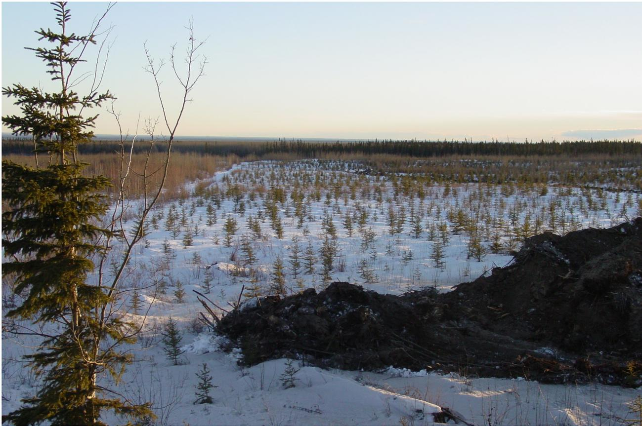
Figure 6. Overview of the landscape beside the Kotcho East gravel pit. The edge of the deposit as indicated by test pits and EM data approximately extends from left to right across the centre of the photo. Note the lack of topographic relief marking the edge of the buried deposit, even though the area has been cleared (seedlings are about a metre high). The dark area at right-centre is a soil stockpile.
