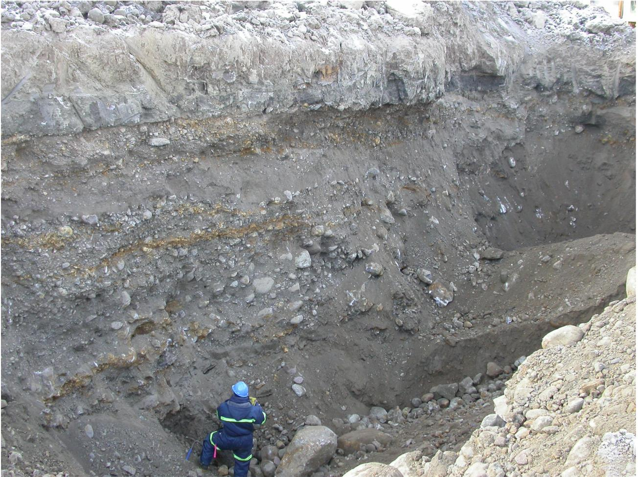
Figure 3. February 2005 exposure in the southwest corner of the Kotcho East gravel pit, operated by EnCana Corporation. Buried gravels in the area are up to several metres thick and the overlying clay-rich sediments are typically 1-2 m, but up to 5 m, thick. The upper part of the overburden has been stripped here and the base of the gravel is below the base of the exposure.
