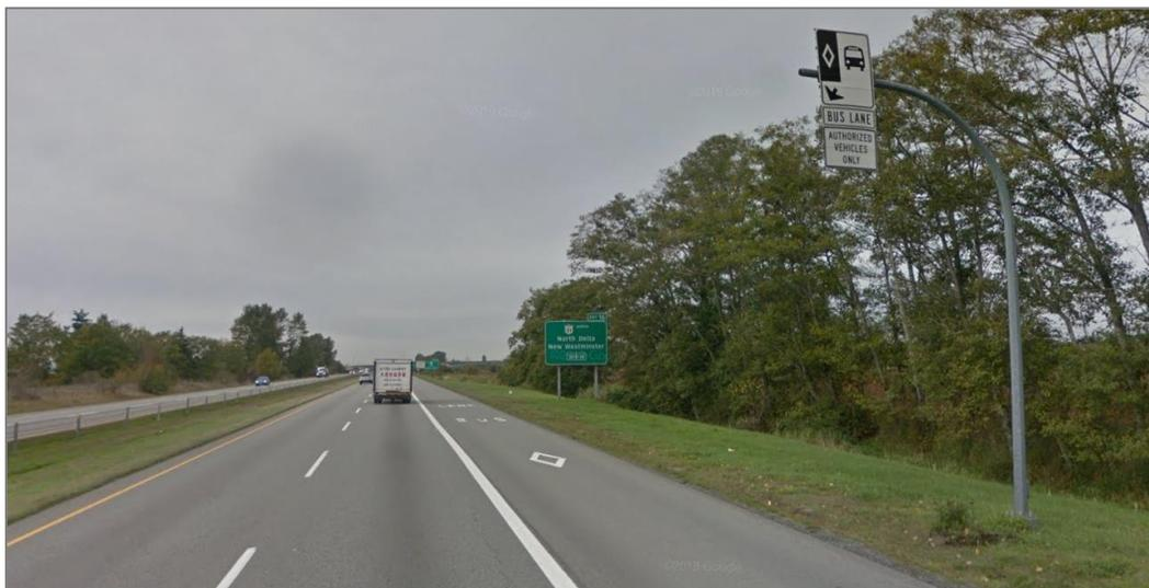
Figure 3.2: Example of a Full-Time Outside Shoulder Bus-on-Shoulder System in Surrey, BC
