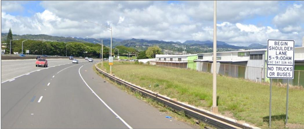
Figure 3.5: Example of an AM Peak Hour Hard Shoulder Running System in Honolulu, Hawaii
