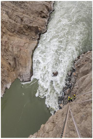
Rock scalers rappel down the 125-metre west canyon slope to manipulate rock at river level.
