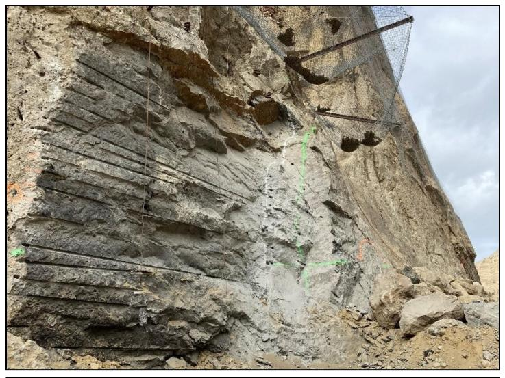
PICTURED: Crews completed drilling to prepare for the second trim blast.
