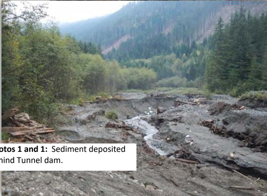
**Photos 1 and 1:** Sediment deposited behind Tunnel dam.
