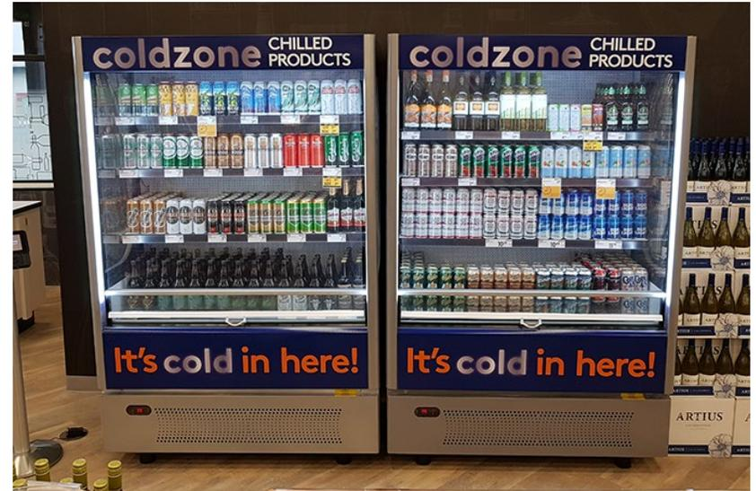
*Open-front coolers at BCLS are equipped with a shade that is drawn at closing time every evening to reduce excessive cooling.*
