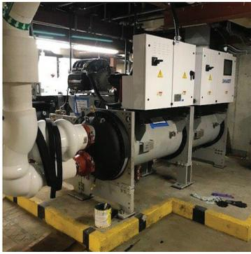
At our Edmonds office building we upgraded the end-of-life chiller system including the installation of variable frequency drives to increase the overall efficiency of the system. The new chillers provide cooling to the building during the summer months and operate 50% more efficiently than the old chillers with an annual electricity savings of about 200,000 kWh.
