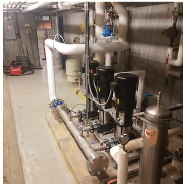
We upgraded the three cold-water booster pumps that were at end-of-life at the Edmonds office building to a new more energy efficient system that can meet the demands of the building as the usage requirement increases and decreases throughout the day. This will save about 100,000 kWh of electricity per year.
