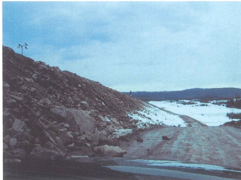
Construction of d/s shell.
