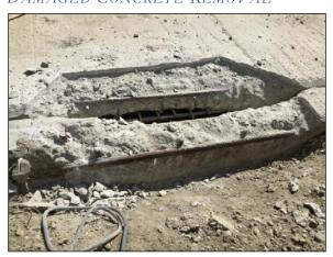
Figure 3: Site preparation in progress – removal of damaged concrete on top of ballast wall and end deck panel. Note saw cut square edges.
