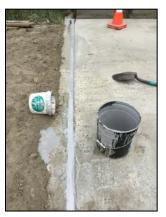
Figure 12: Paraseal sealant placed at gap between ballast wall and concrete deck subsequent to concrete repair works.
