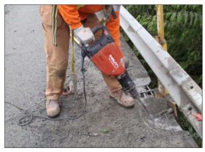
Figure 4: Mechanical removal of damaged concrete with a chipping hammer
