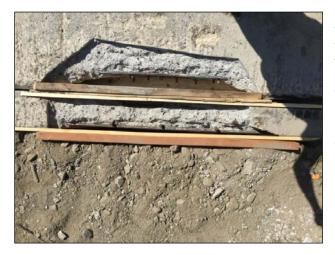
Figure 7: Formwork placed, subsequent to removal of damaged concrete, to contain grout for ballast wall and deck panel repair.
