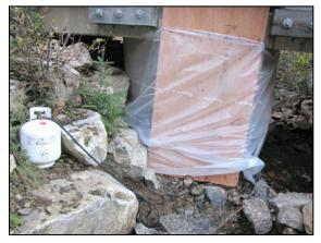
Figure 9: Makeshift tent used with a Tiger Torch to provide heat in cold temperatures to improve grout curing conditions for the repair site. This method is known as 'hoarding'.
