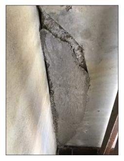
Figure 8: Formwork on underside of deck panel removed showing grout patch inadequately tamped along the edge of the formwork; see Figure 7 for additional repair.
