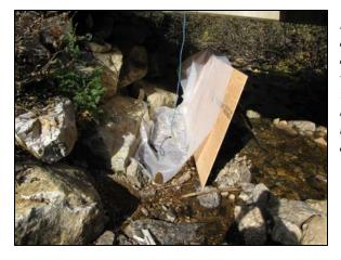
Figure 2: Example of a collection system for containing debris and waste for the work site. This could be improved by using a larger tarp to better ensure all debris is captured.
