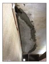
Figure 11: Additional grout patch being placed into bottom of a deck panel, adjacent to a ballast wall, to fill voids from initial unconsolidated repair work to obtain original deck dimensions
