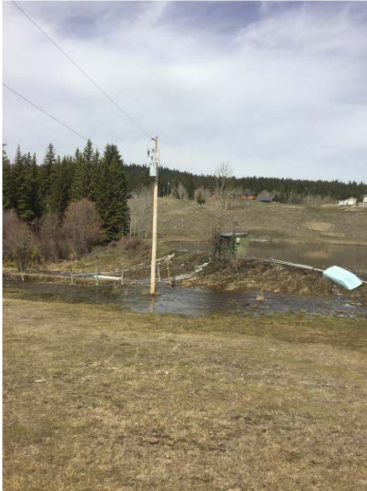
Photo 3: Overtopping and erosion of the Valley Pond (Upper) Dam embankment
