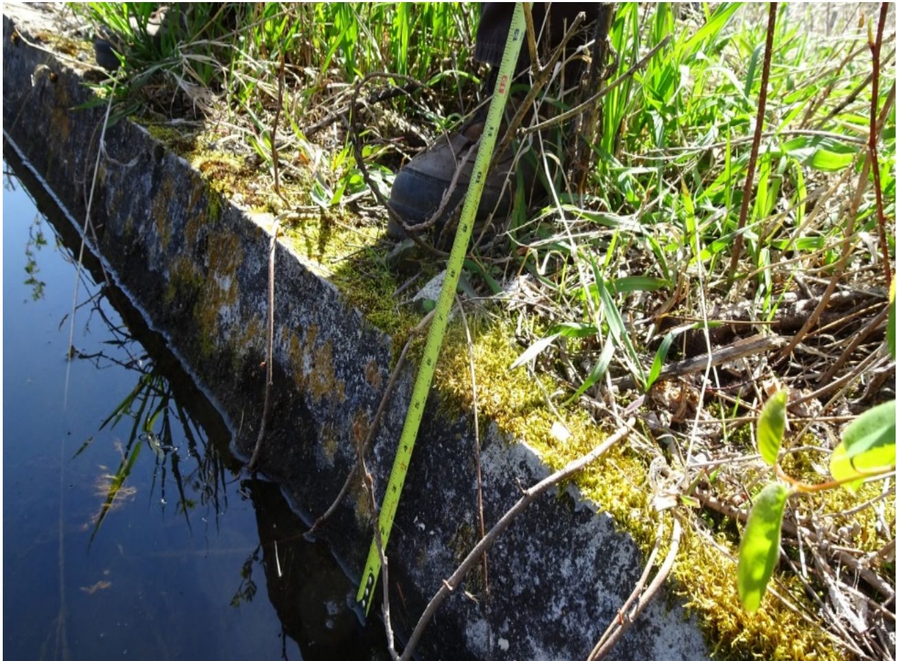
Photo 7: Three-inch freeboard left on the Park Rill dam at the highest water level
