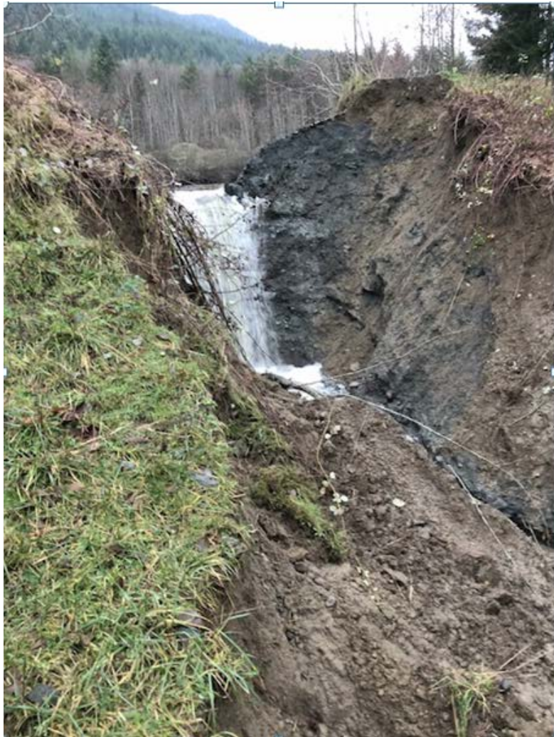
Photo 1: Stable breach on dam on Dalzell Creek
