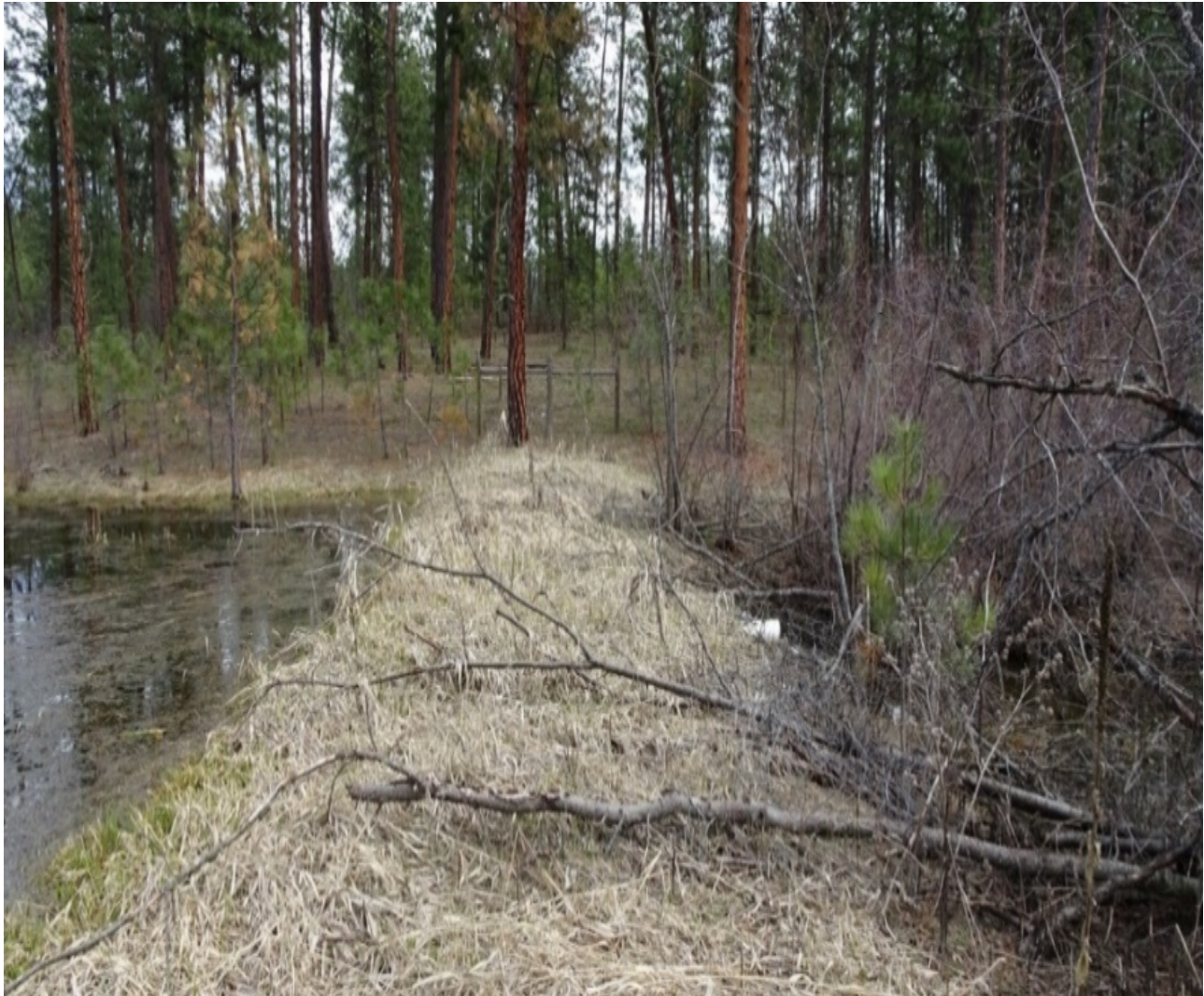
Photo 4: Bubna Slough dam near overtopping from high water level in reservoir
