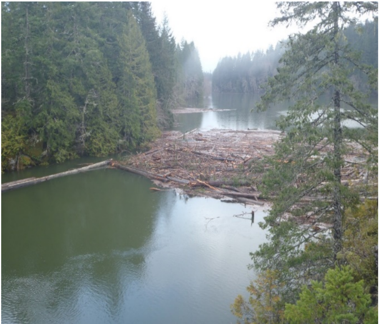
Photo 11: Log debris held by free floating log boom located upstream from the South Fork Dam
