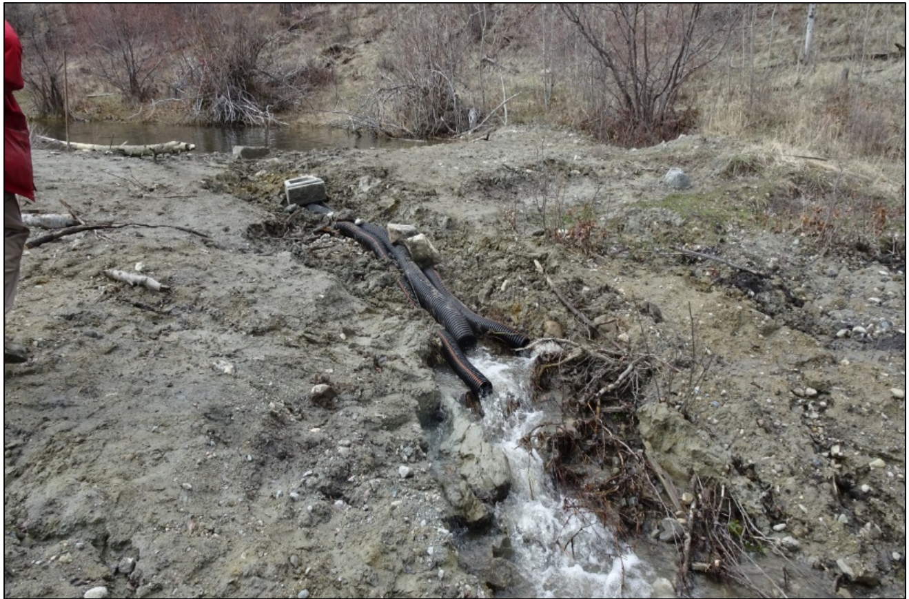
Photo 8: Siphoning of the reservoir also caused erosion of the Saltgrass Pond dam
