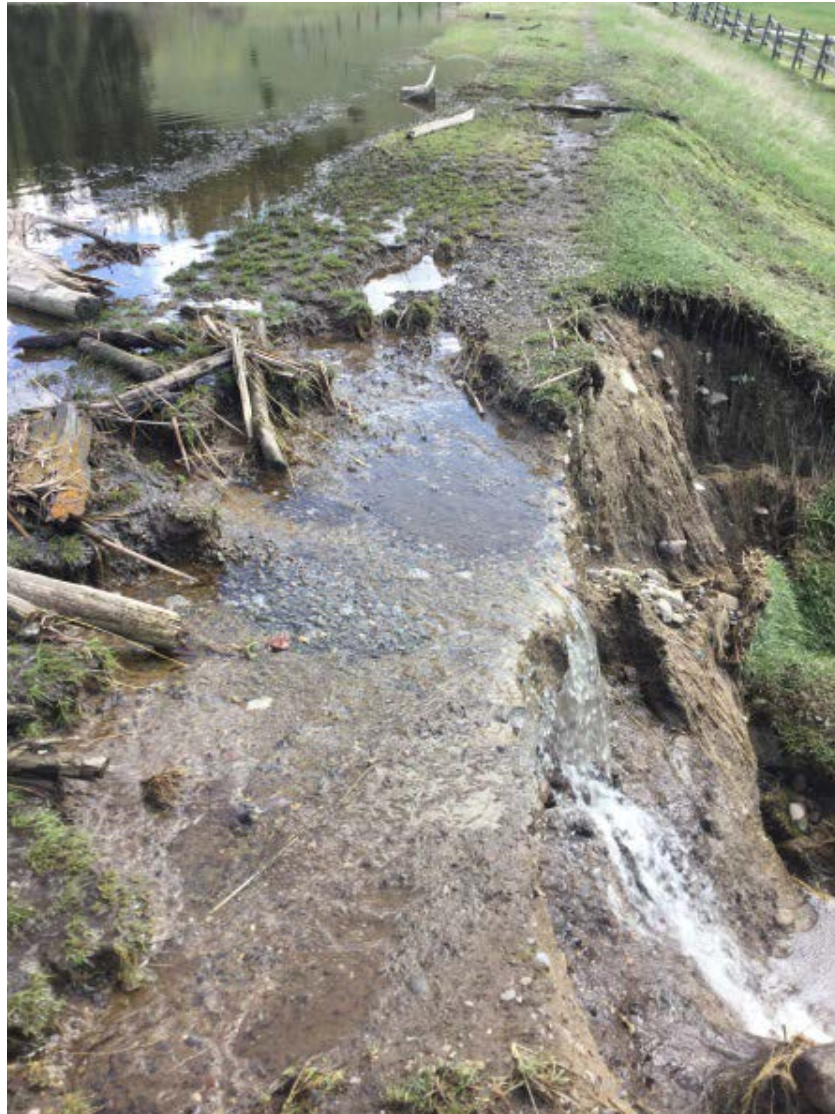
Photo 2: Unknown dam near Riske Creek overtopping.
