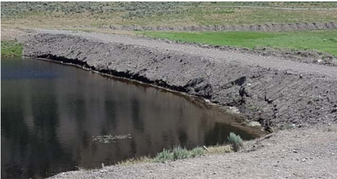
Photo 10: Upstream slope of Frank Lake dam showing signs of slumping
