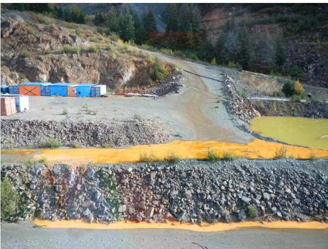
Photo 5 Exfiltration pond. Note overflow of mine portal water.
