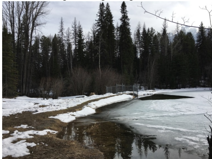
Photo 4: High lake level at Tie Lake Dam, resulting in loss of freeboard
