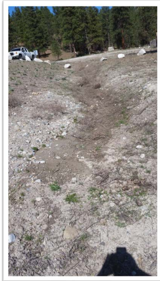
Photo 2: Seepage track on the downstream side of the left abutment of Aeneas Lake Dam
