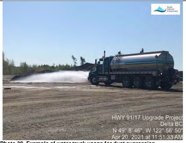
Photo 30. Example of water truck usage for dust suppression.
