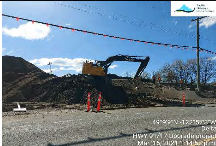
Photo 3. Preload removal ongoing at the L325(C).
