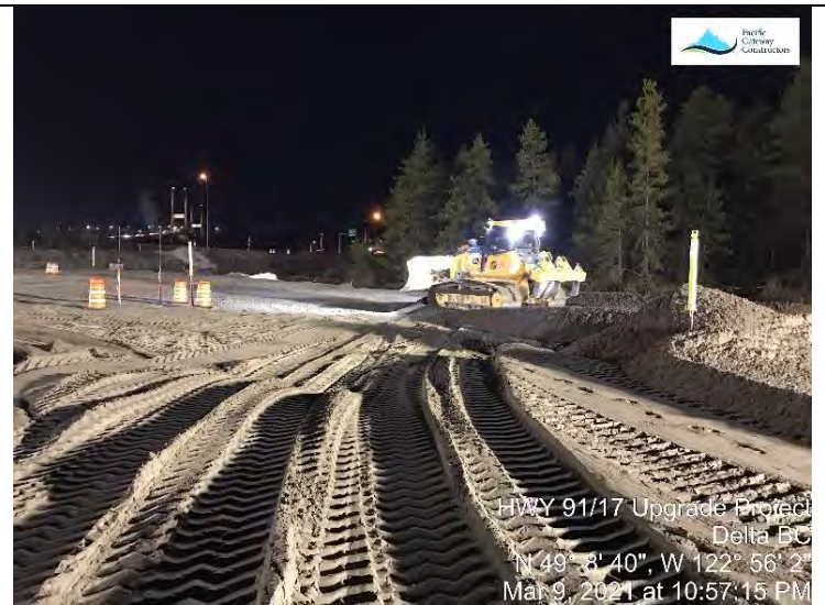
Photo 24. Placement of preload sand continued at the L2300 (G).
