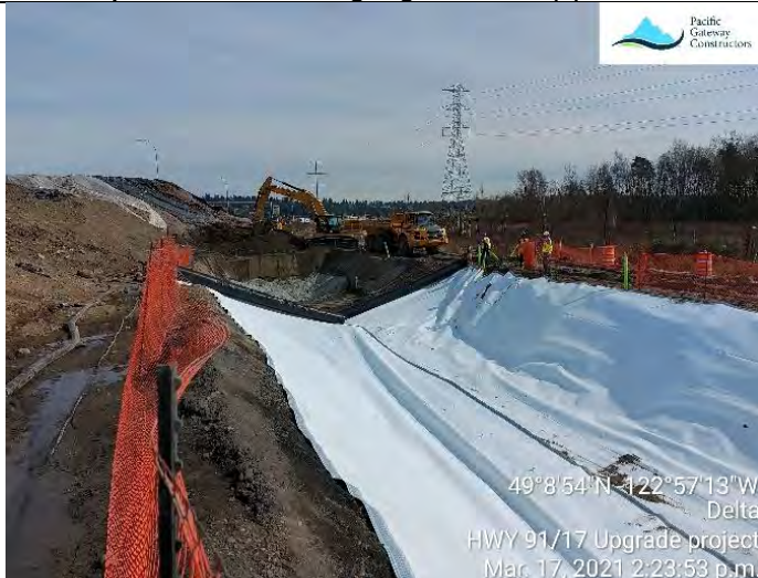
Photo 13. General view of contaminated soil placement at L550 (E).
