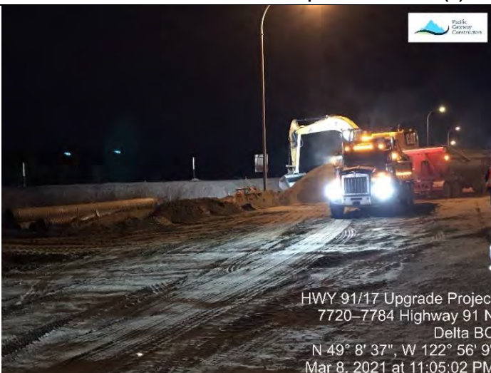
Photo 15. Offloading of preload sand from Hwy 99 at the L1400 (F).
