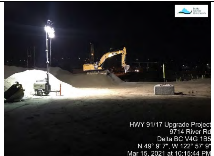
Photo 2. Removal of preload sand continued at the L295 (C).
