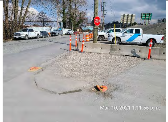
Photo 32. Damaged CB inserts on River Road West (C).
