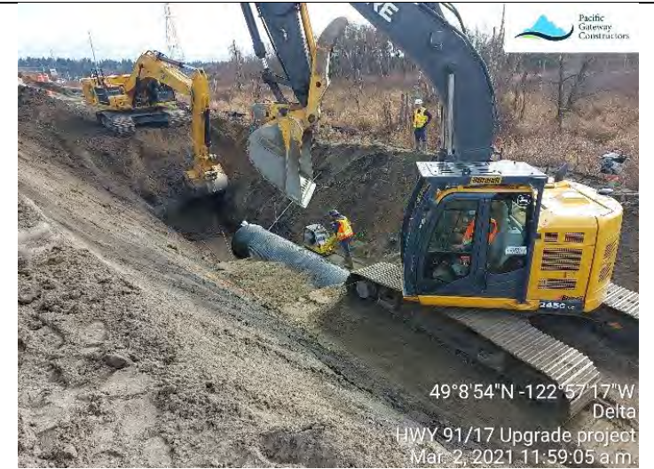
Photo 10. Culvert installation ongoing at the L550 (E)..
