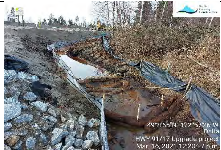
Photo 8. ESC measures are being installed in the L400 ditch (B).
