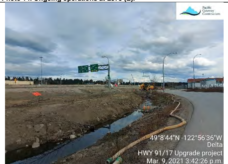
Photo 16. Area F ditch rip rap removed at the L1145 (F).
