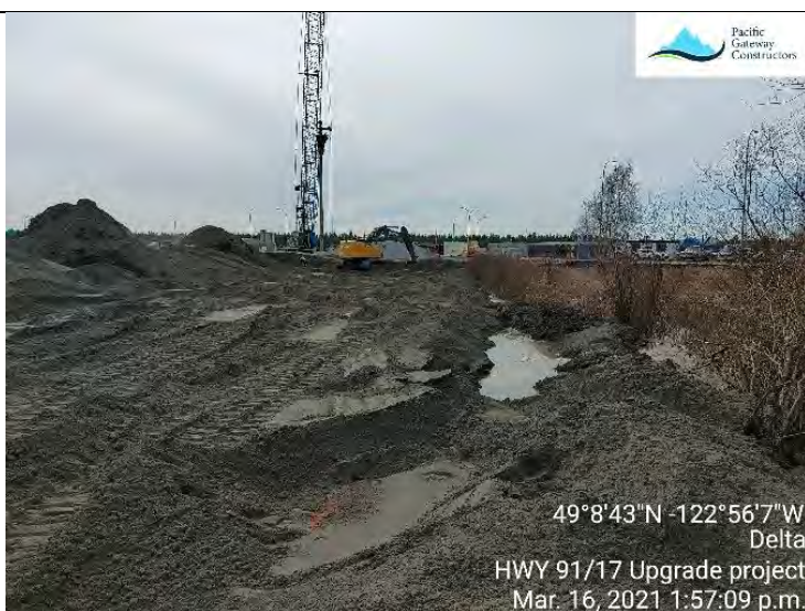
Photo 27. Placing sand preload at the L2300 (G).
