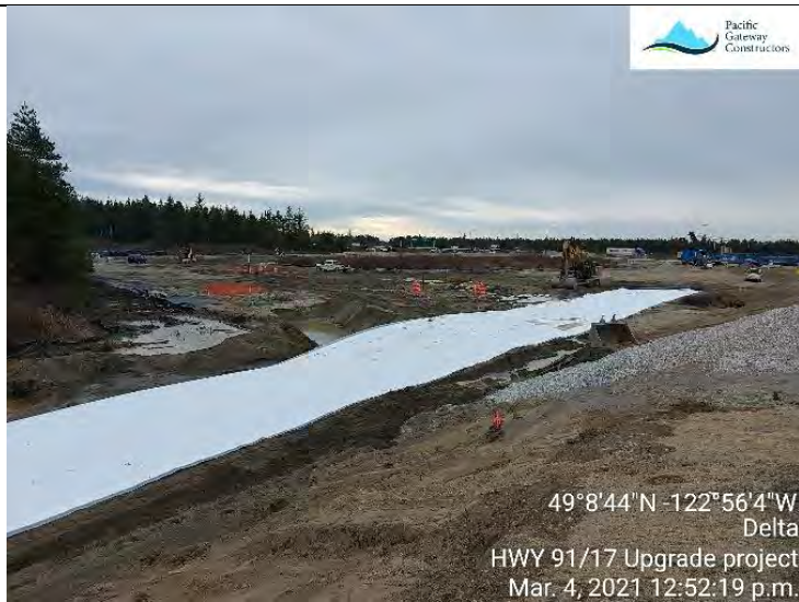
Photo 23. Installing the geomembrane at the L2300 (G).
