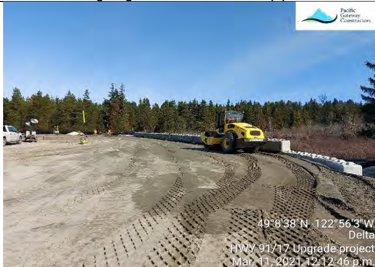
Photo 25. Preload placement ongoing at the L2300 (G).
