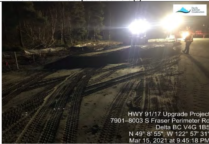
Photo 7. Repairs done to subgrade settlement issues over catch basin pipes at the L100 (B).
