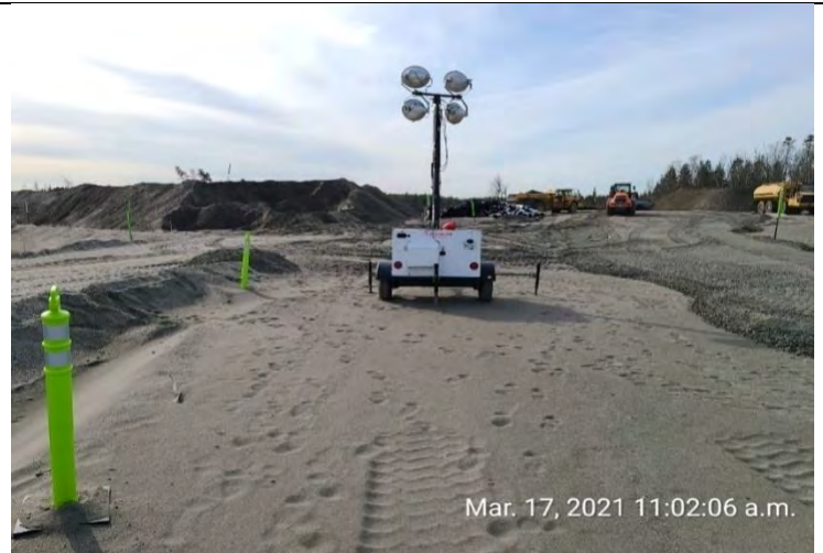
Photo 36. Drip trays are lacking throughout the Site, particularly for light stands
