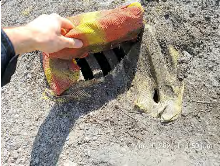
Photo 31. Damaged CB inserts on River Road West (C).
