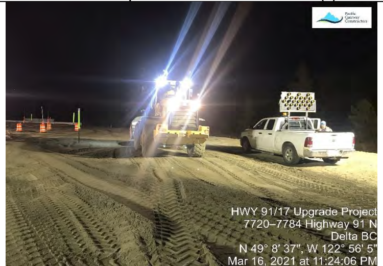
Photo 26. Placement and compaction of preload sand continued at the L2300 (G).
