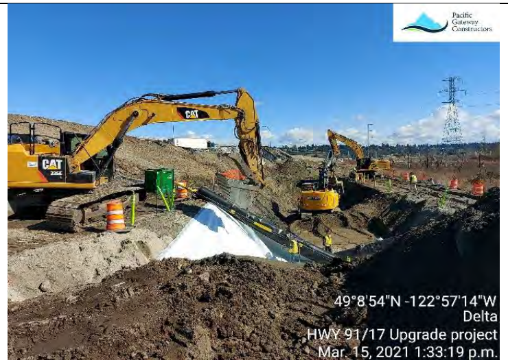
Photo 12. Culvert pipe run installation ongoing at the L550 (E).
