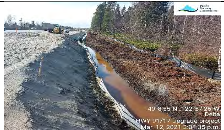
Photo 6. Ditch silt fence ESC installed at the L400 (B).
