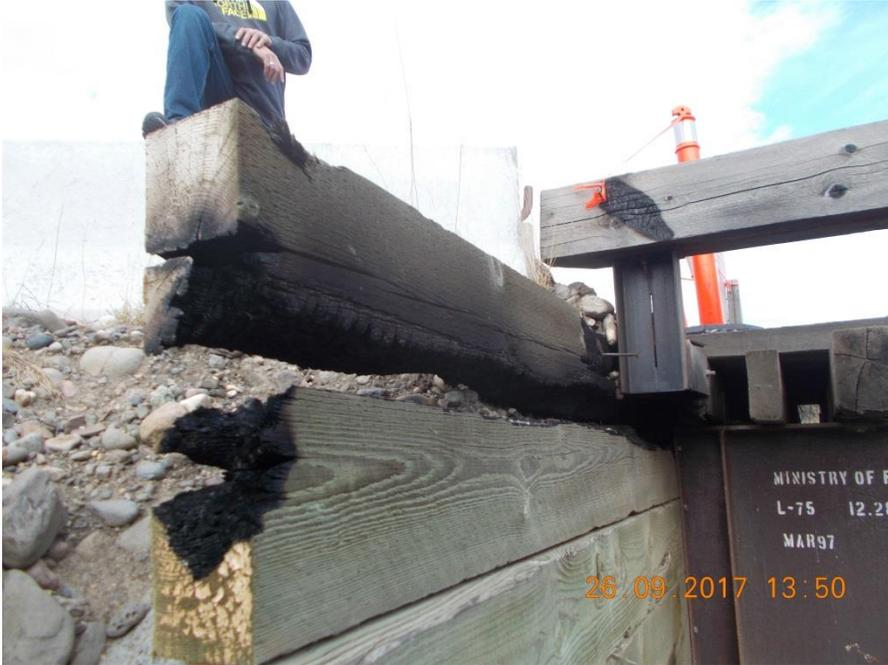
Photo 1a - Slight damage to ballast wall, curb, and end of one tie
