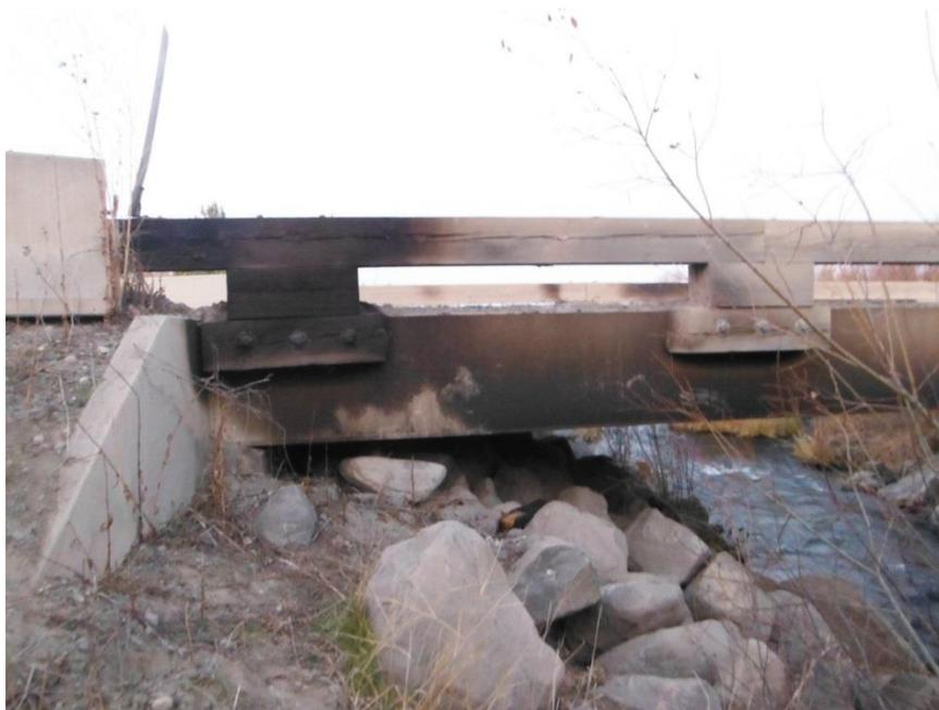
Photo 5b - Fire evidence seen on side of bridge
