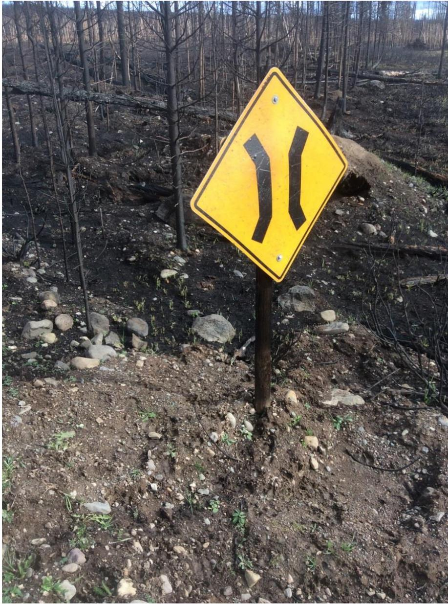
Photo 6 - "Bridge Ahead" sign: fire damaged post
