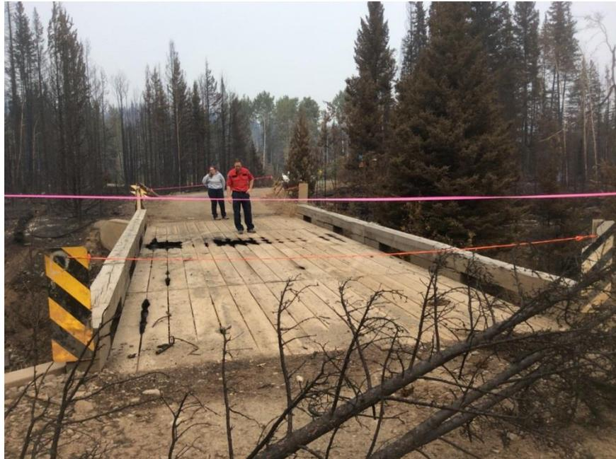
Photo 3a - Timber deck partially burnt
