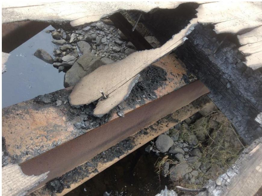
Photo 3b - Close-up view of burnt deck section
