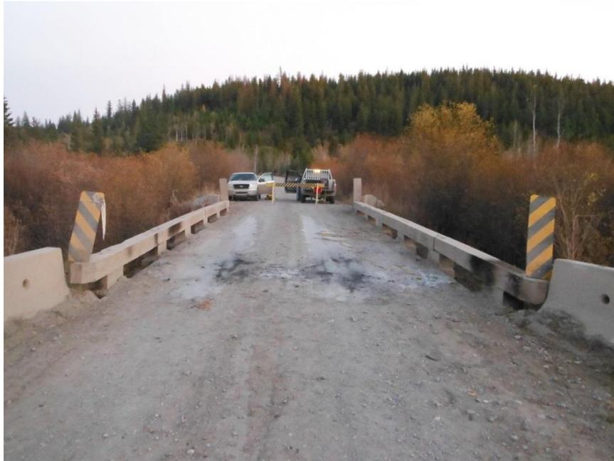
Photo 5a - Fire evidence seen at top of bridge
