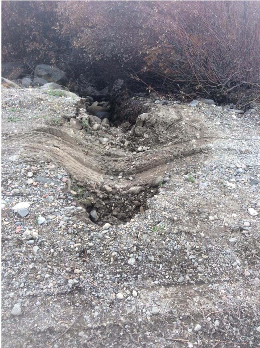
Photo 7a - Roadway collapse due to melted plastic culvert
