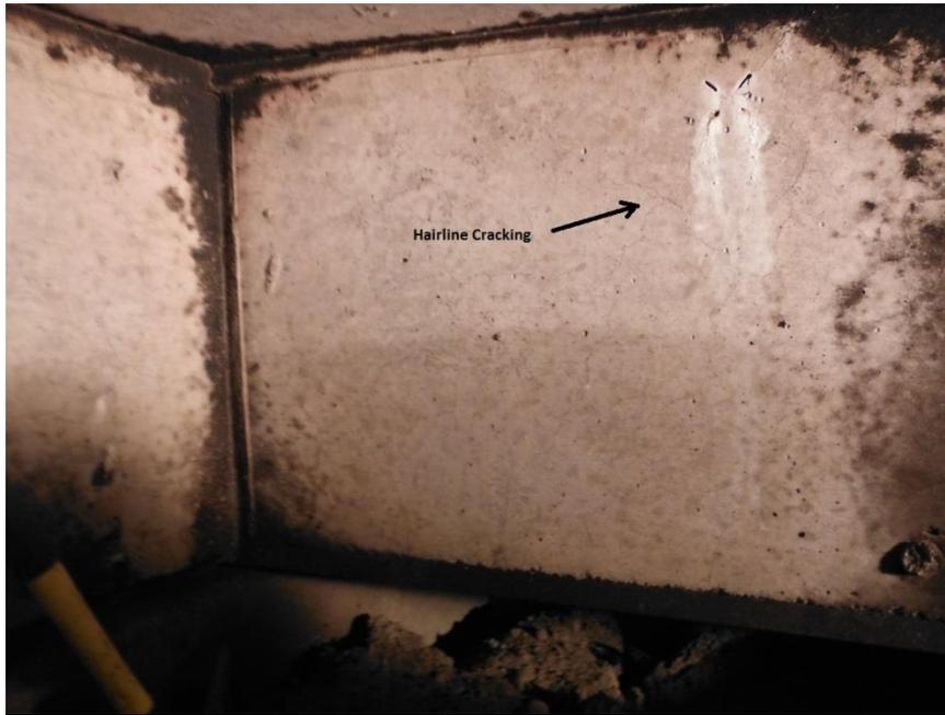
Photo 5e - Hairline cracking on side of girder (top right quadrant of photo)
