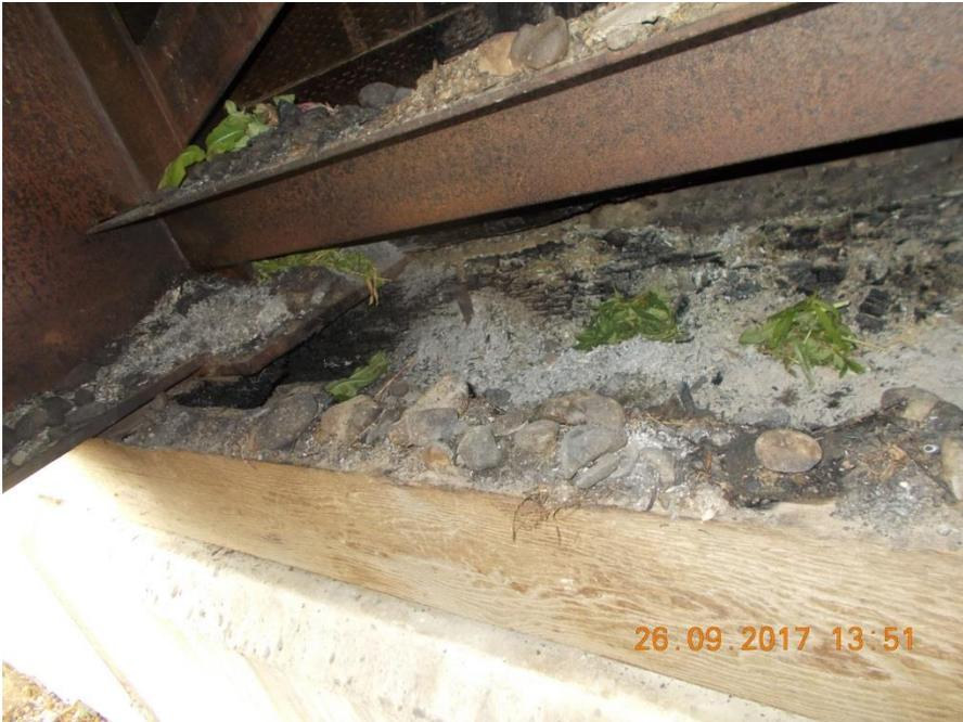
Photo 1b - Cap burnt between girders and under bearing plate
