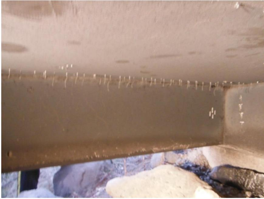
Photo 5c - Melted rebar chairs on deck soffit
