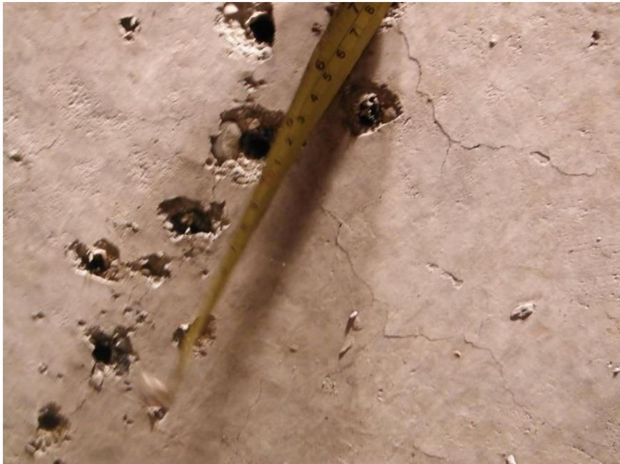
Photo 5d - Concrete spalling and cracking (presumably from fire)
