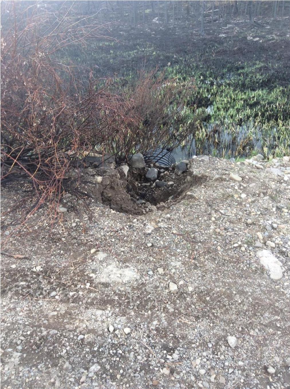
Photo 7c - Roadway collapse near inlet/outlet due to melted plastic culvert
