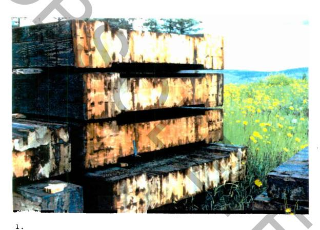
Glued-laminated girders that were taken out of service, as a result of consultant's recommendations, due to observed cracks.
