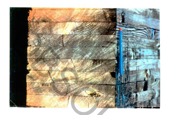
The bridge girders were cut into 20.0 feet long segments for ease of transportation. It is interesting to observe the extent of the surface checking. These surface checks would certainly not reduce the capacity of the girder section!
