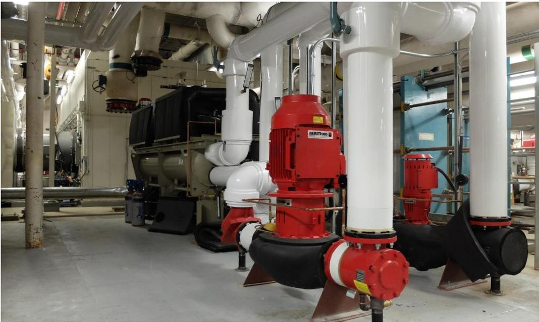
Heat recovery chiller and pumps installed at Vancouver General Hospital.
