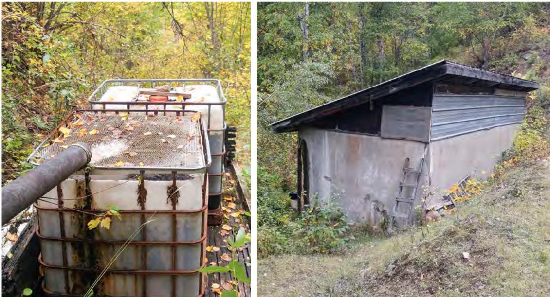
A small water system in the West Kootenays of BC's interior. Diverted creek water passes through a screened collection system (left) to remove sticks, leaves, and debris before entering the storage reservoir (right). Water is delivered to homes on the system by gravity with no further treatment. The water system has been on a boil water notice for more than 30 years. Untreated drinking water is the most common cited reason for drinking water advisories in BC.
