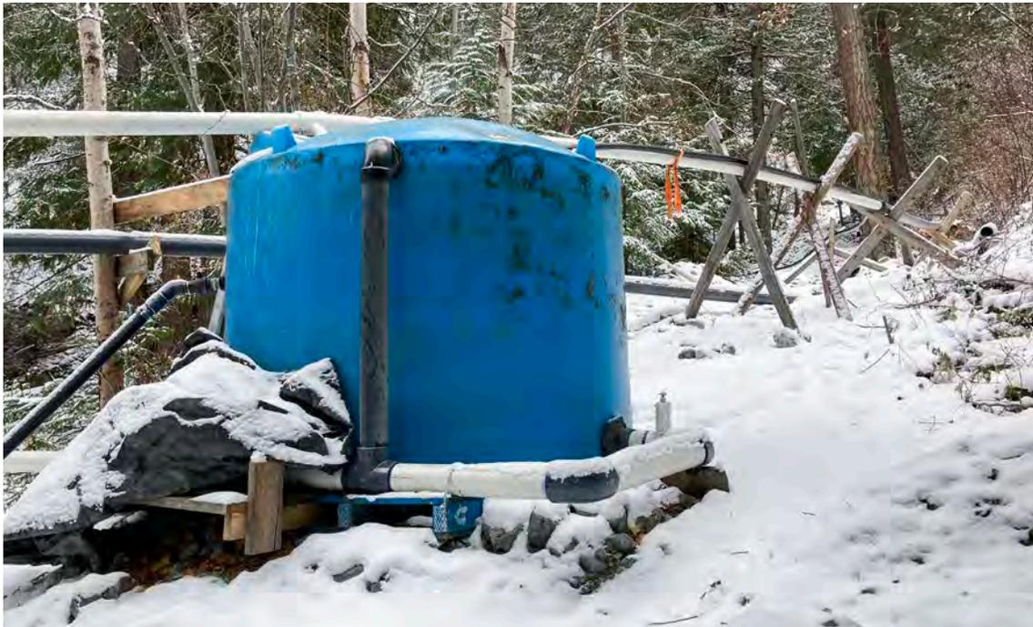
Overland piping and emergency storage tank at Gladwin after damages from debris flow.
