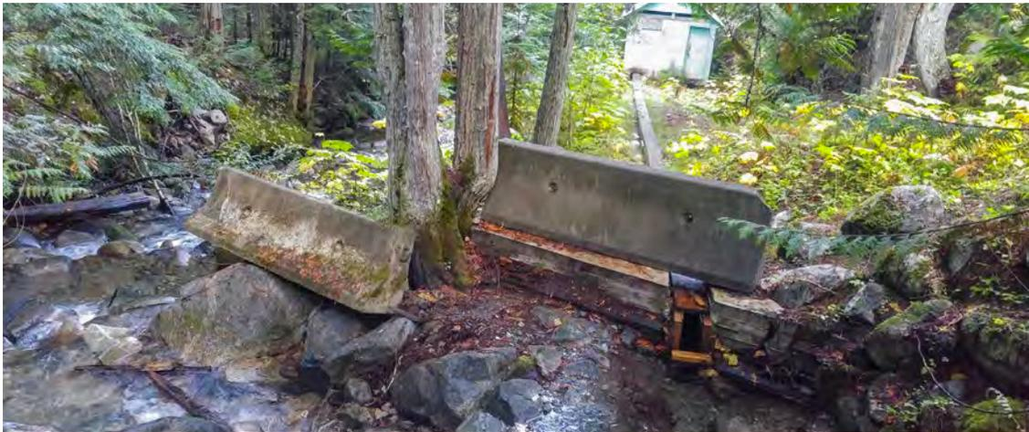
**Sandy Creek Water Users' Community near Nelson, BC.** The intake of Sandy Creek leads to a concrete reservoir. The system supplies 83 connections via gravity but has no treatment, and a long-term boil water notice has remained in place for more than three decades.
