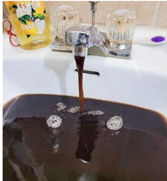
A customer supplied by the Town of Osoyoos water system experienced a slug of manganese deposits in their drinking water after a nearby hydrant was disturbed. Physical disturbances to a distribution system can cause the release of manganese deposits from pipes. In June 2023, the Town of Osoyoos was granted \$9 million to assist with water infrastructure projects to improve drinking water quality.
