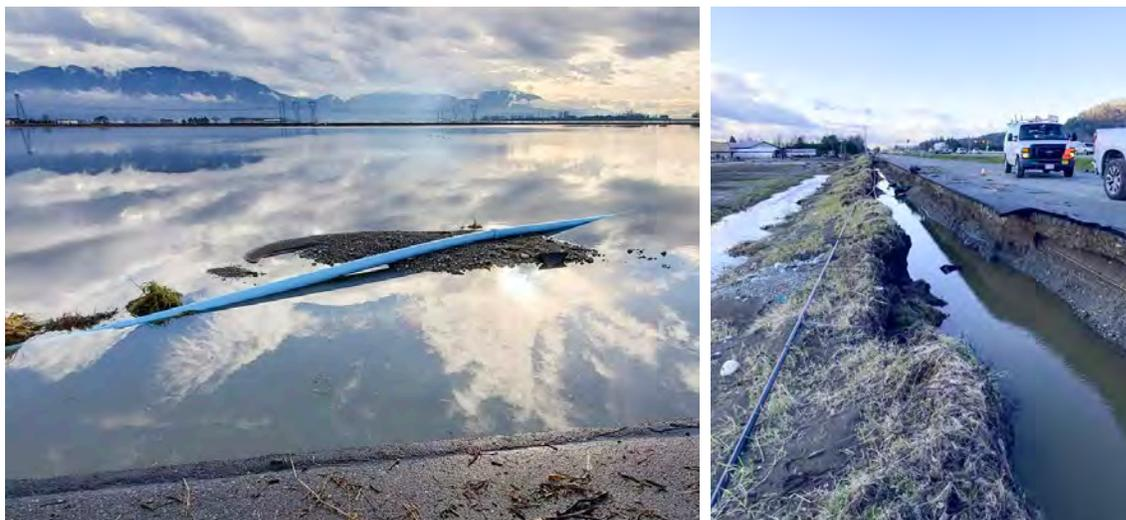
In the aftermath of the flood, damages to the distribution system became visible in Sumas Prairie. (Left) A broken six-inch water main in Sumas Prairie after the flood. (Right) City of Abbotsford staff worked to assess the damages and estimate the replacement work needed for the water system within the isolated zone of the distribution network.
