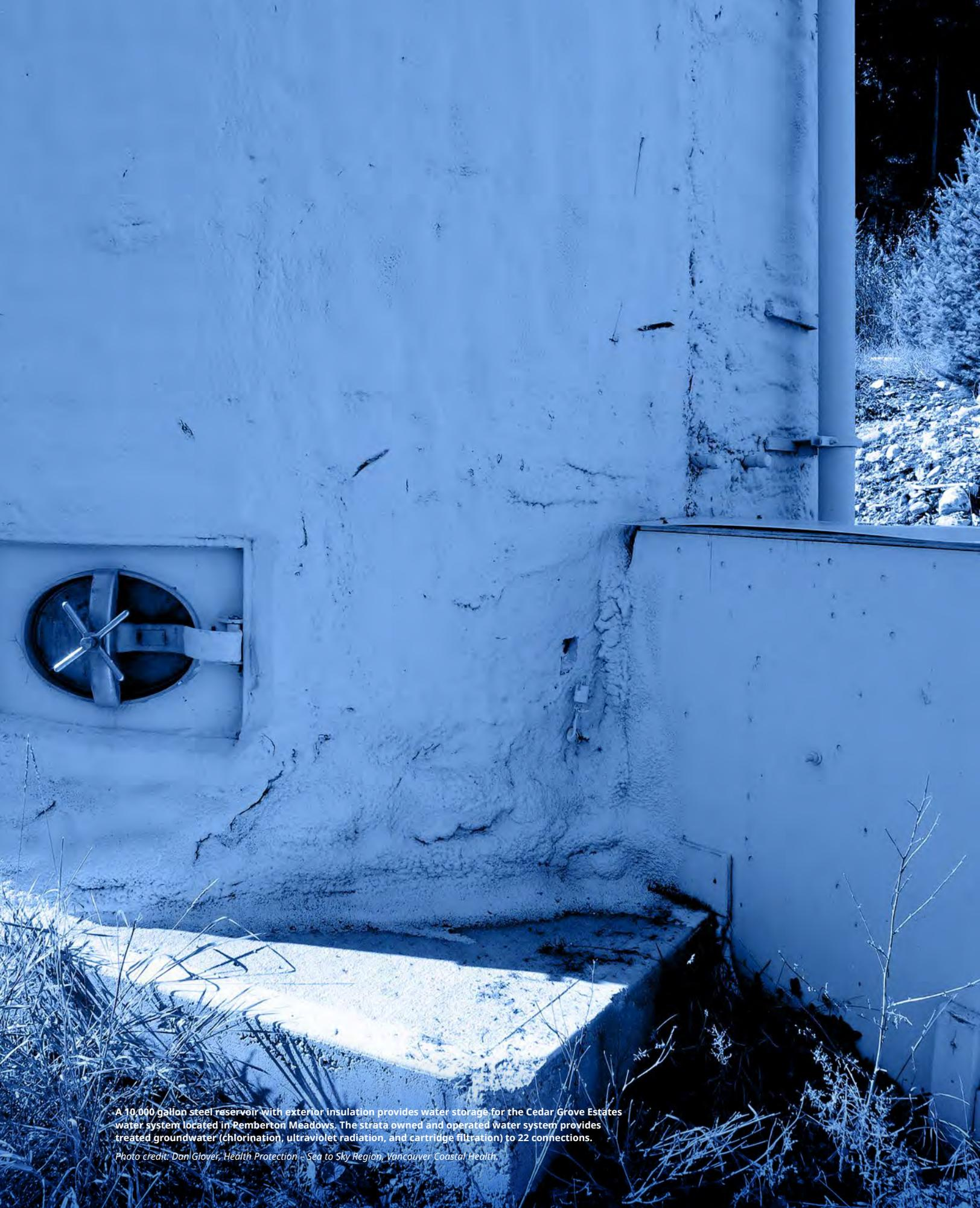
A 10,000 gallon steel reservoir with exterior insulation provides water storage for the Cedar Grove Estates water system located in Pemberton Meadows. The strata owned and operated water system provides treated groundwater (chlorination, ultraviolet radiation, and cartridge filtration) to 22 connections.
