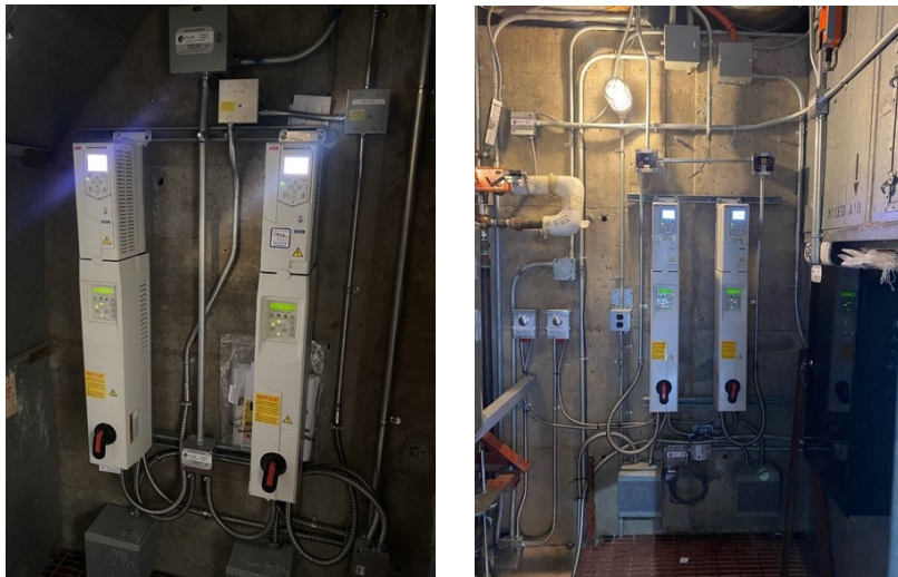
Figure 2 - Two VFD mounted in a mechanical room
