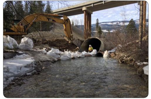
Large bags filled with gravel were used to divert the creek temporarily into a small culvert (right of the worker), so the original large culvert could be removed.
