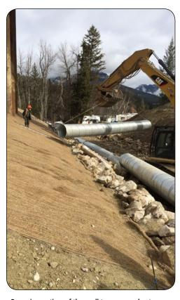
Removing sections of the small temporary culvert, once rip rap was in place to shore up the creek.
