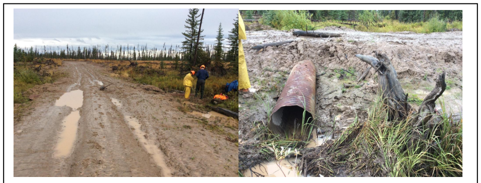
Figure 9: Stream Crossing with High Sediment Loads
