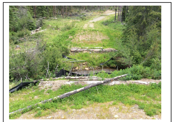
Figure 8: Well Managed Deactivated Stream Crossing
