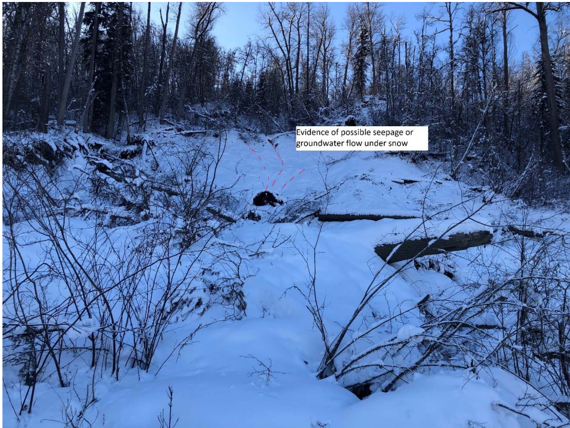
Photo 3: Landslide mass above Quesnel Hydraulic Road at Slide B indicating possible surface groundwater or formation seepage discharge from the headscarp
