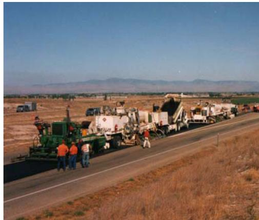
A typical two-stage milling process uses the following equipment in a continuous train:
