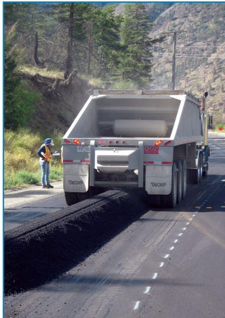
Since the plant operates continuously, an adequate truck capacity must be ensured. Otherwise, the asphalt production process risks being backed up waiting for trucks or the paving crew to catch up. This, in turn, reduces plant efficiency.
