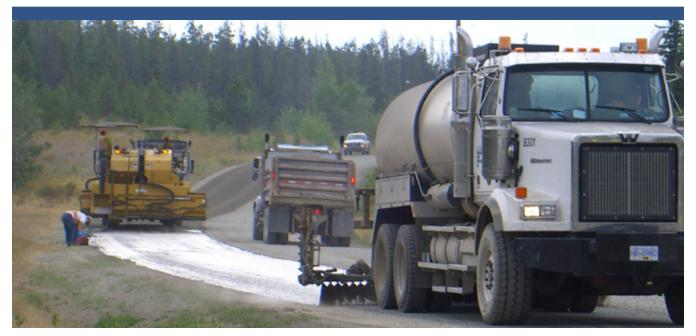
Seal Coating is the application of a special protective wearing surface to an existing pavement or gravel base.
