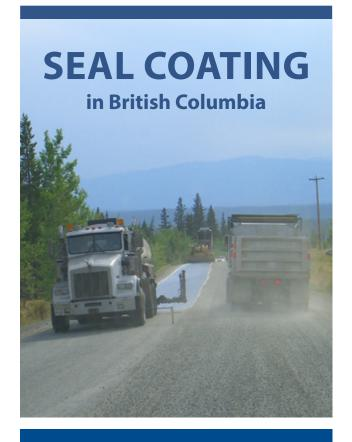
Seal Coating is the application of a special protective wearing surface to an existing pavement or gravel base.
